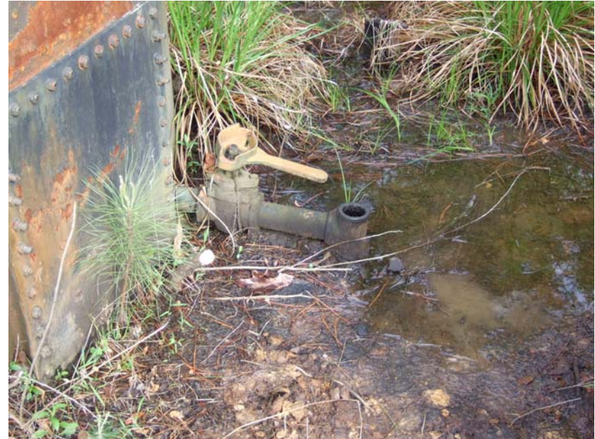
Site Name: Quality Petroleum, Inc.-Hoffman, et al. Project No.: E06614 Photo No.: 0209 Direction: Down Contract No. Date: 04/05/2008 Time: 9:38:00 AM Photographer/Witness: Sekerka, Robert/Johnson, Colin Description: E06614: Oil saturated soil surrounding valve on AST2.
