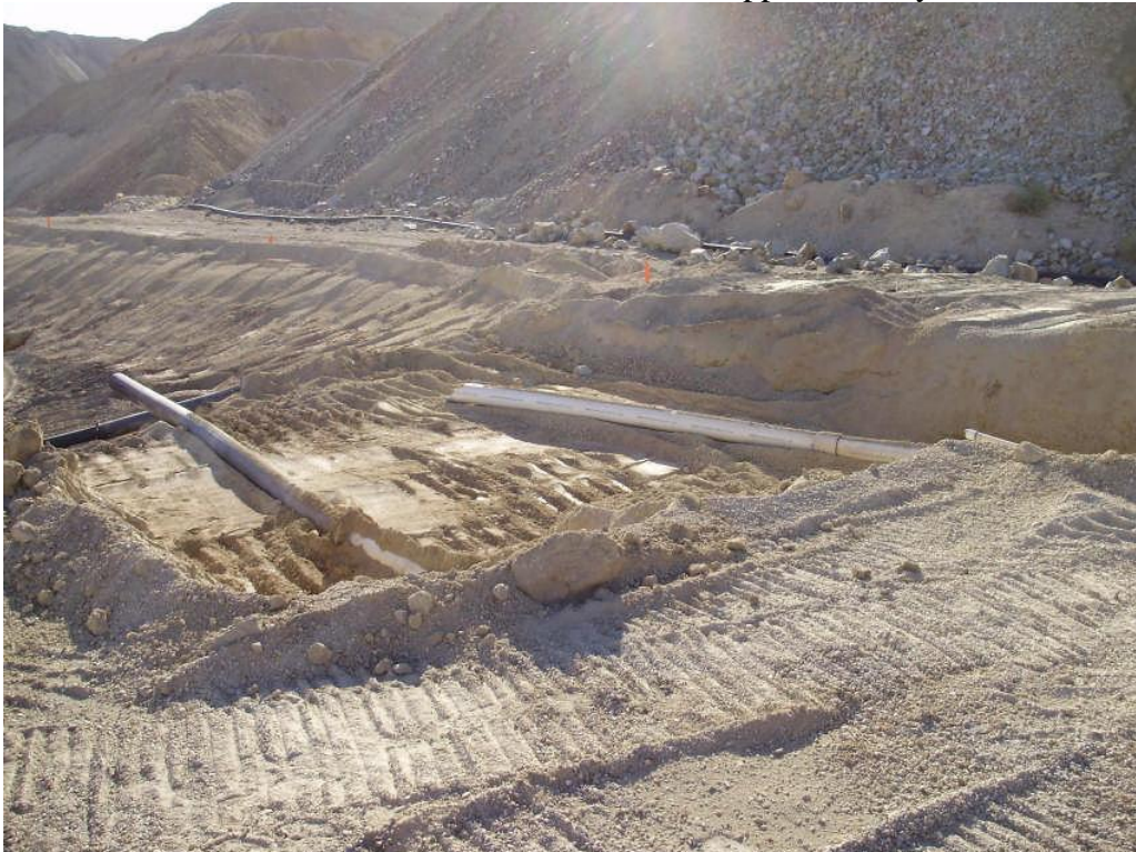
Photo 4: Piping connecting the Old Raffinate Pond to vaults.
