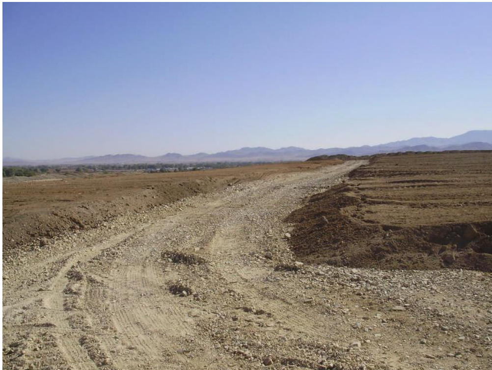
Photo 6: Bioremediation cells with soil excavated from the Old Raffinate Pond.
