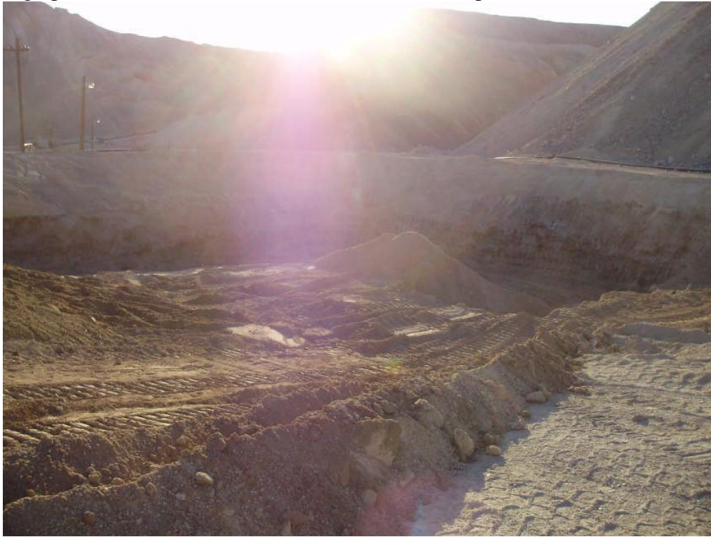
Photo 5: Old Raffinate Pond excavation at approximately 15 feet.
