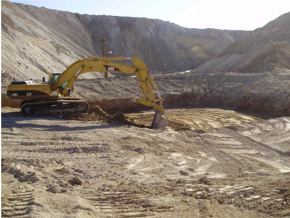
Photo 3: Old Raffinate Pond excavation at approximately 5 feet.
