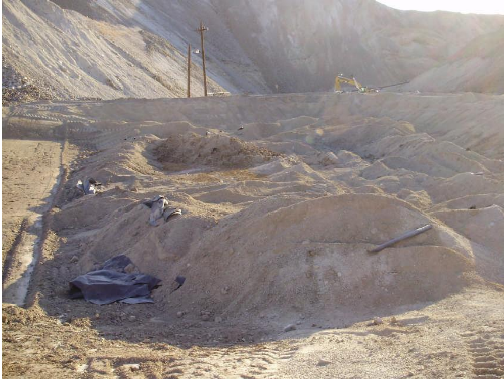
Photo 1: Old Raffinate Pond prior to excavation after liner removal.
