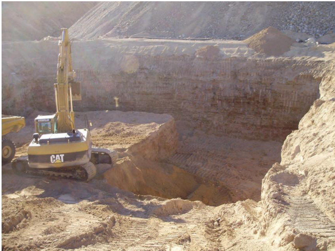
Photo 6: Old Raffinate Pond during excavation to approximately 23 feet.
