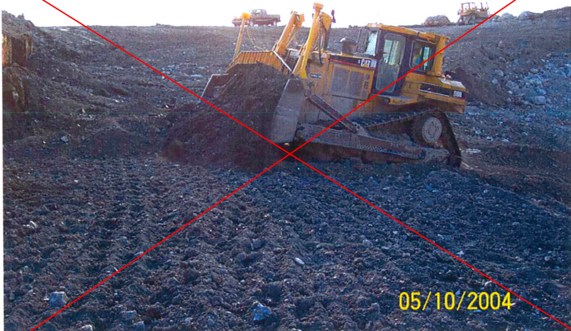
Photo # 23 – Looking west. Beaver placing structural fill on Lift 11.
