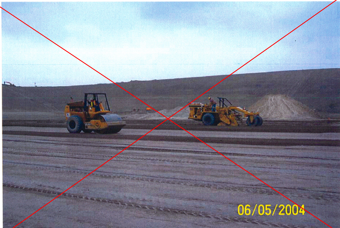
Photo # 19 – Looking southwest. Rototilling and sealing Lift 4.
