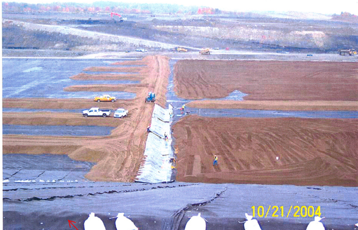
Photo #47– Looking north, temporary Intracell berm installation
