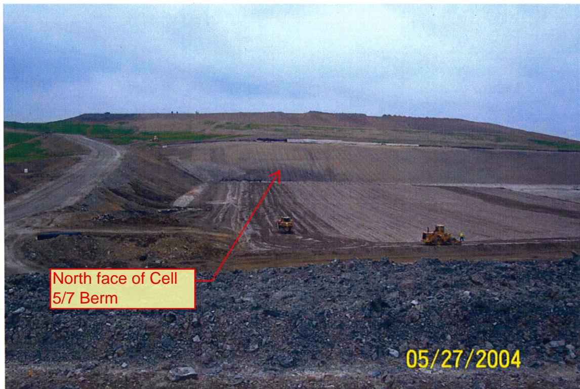
Photo # 10 – Looking south. Recompacted soil liner Lift 1 surface scarifying.
