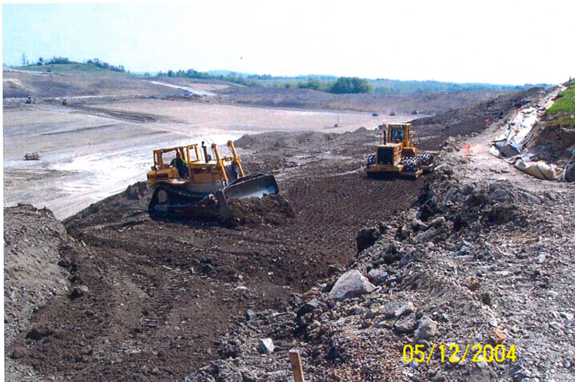
Photo # 24 – Looking northeast. Placing and compacting Structural Fill Lift 2.
