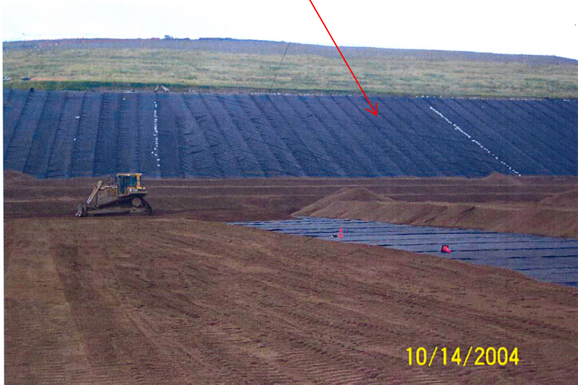
Photo #46 – 12" granular drainage material placement.
