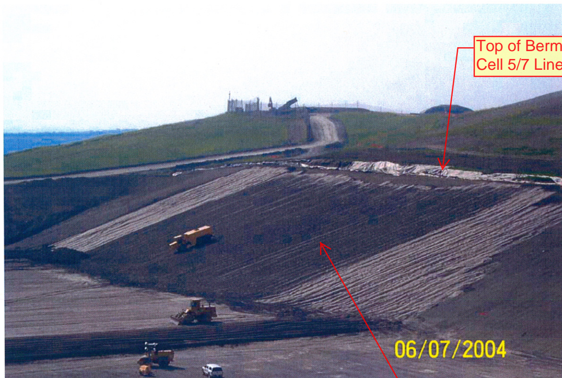
Photo # 20 - Looking southeast. Lift 1 south slope watering.
