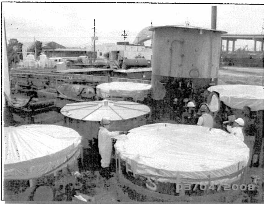
Photograph 11 : Installing 6 mil poly sheeting covers over tank bottoms.
