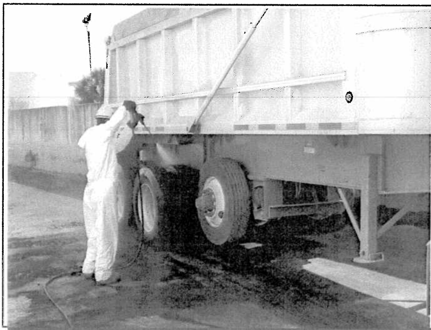
Photograph 14: Pressure washing truck tires before leaving site.
