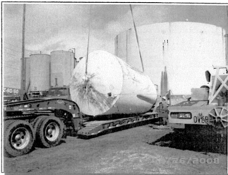
Photograph 7: Loading Tank 109 for transport to Berman Brothers Recycling.
