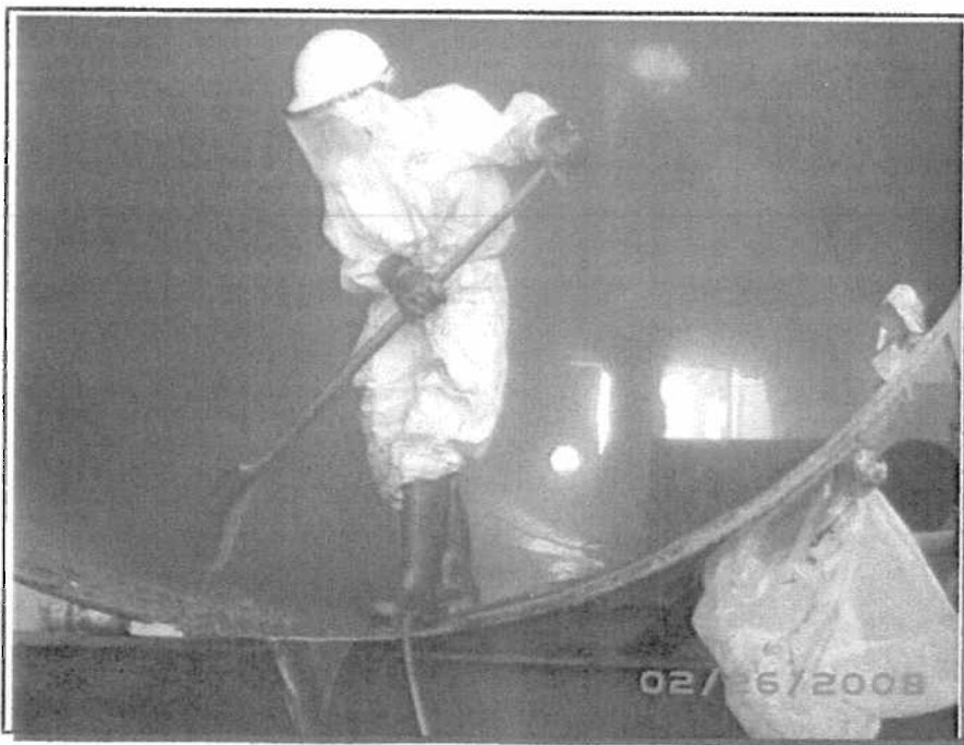
Photograph 6: Pressure washing and removing sludge inside Tank 101.
