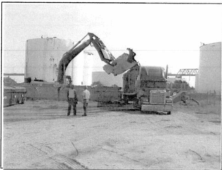
Photograph 18 : Loading tank steel for recycling.
