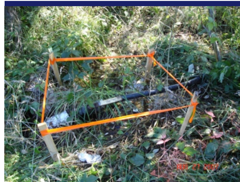
Photo 31 High visibility flagging around residential water line.
