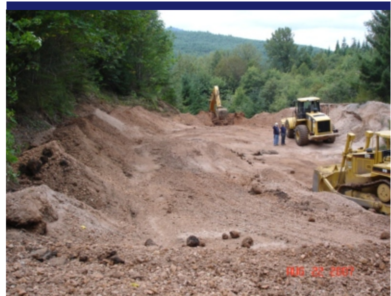
Photo 2 Moving tailings from Main Tailings Pile - West slope up slope.
