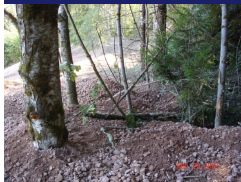
Photo 19 Keying tailings into top of Main Tailings Pile - East slope.
