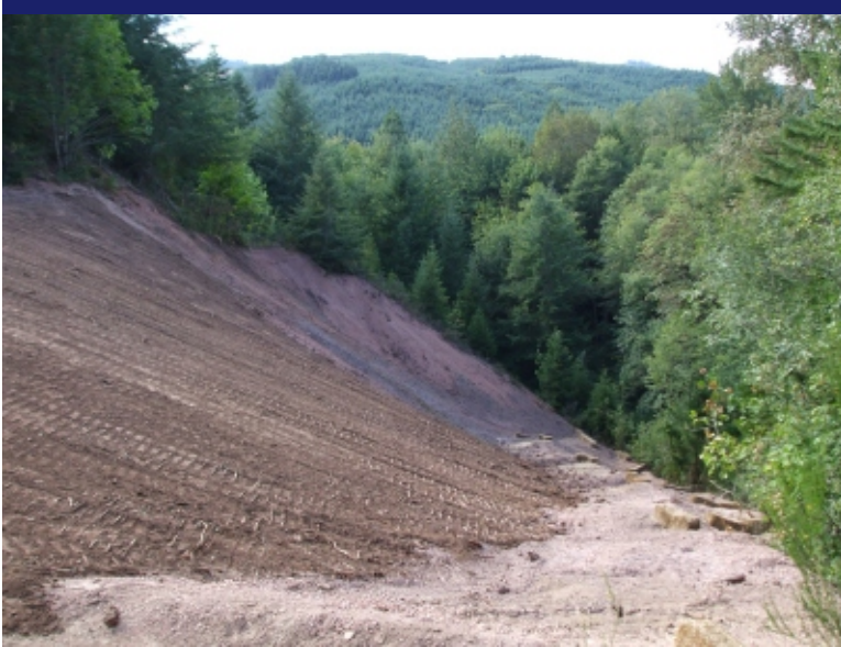
Photo 5 Main Tailings Pile - West slope with soil cap.
