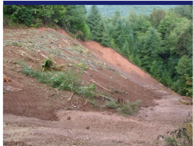
Photo 11 Main Tailing Pile - West slope showing soil cap with woody debris on surface.
