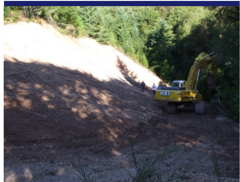
Photo 4 Main Tailings Pile - West slope excavator making water bars at
