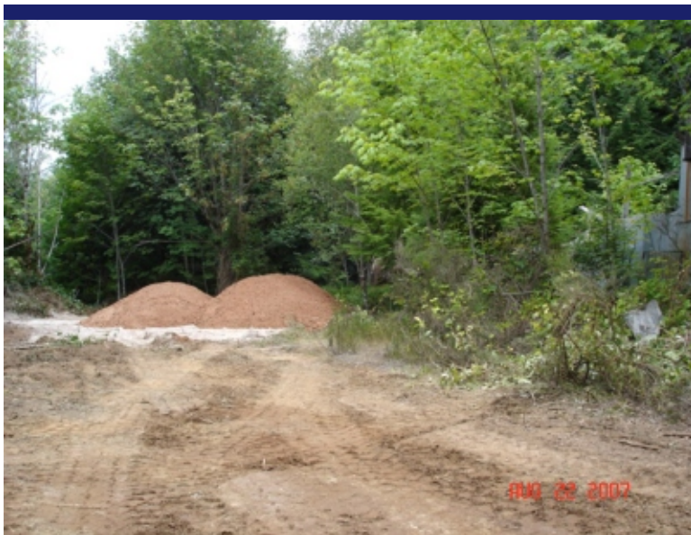
Photo 16 Moving tailings from Main Tailings Piles to New Furnace Area for capping.
