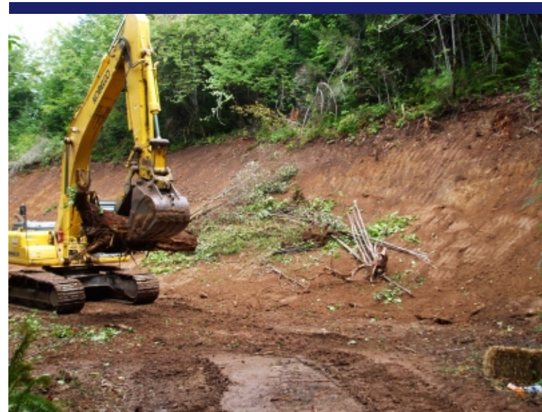
Photo 53 South of New Furnace - Slope reconstruction after fill material removal.
