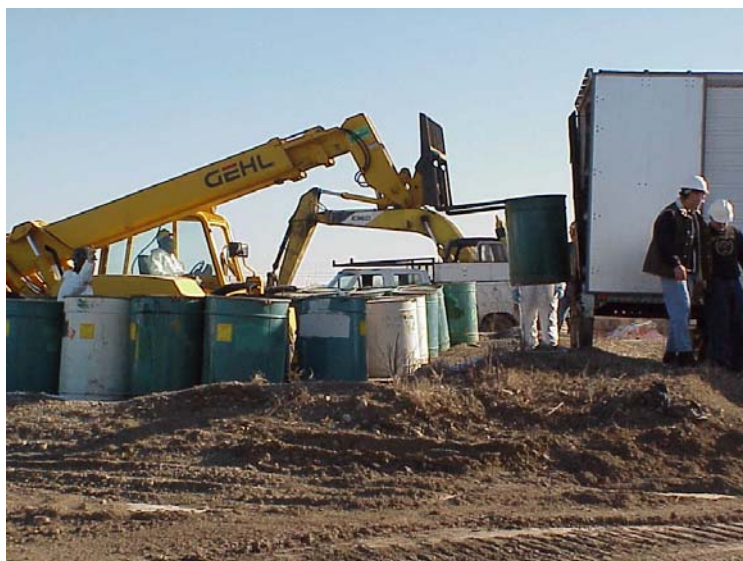
View of hazardous waste drums containing flammable liquid being loaded for off-site disposal.
