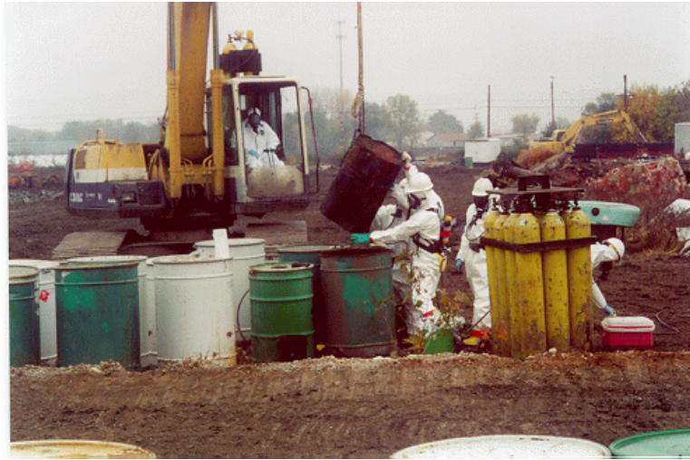
View of VDRAG contractors overpacking an excavated and intact waste drum.
