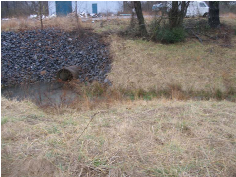
Photo 4: East Drainage Ditch showing 48" Storm Bypass Pipe @ Olin Area.
