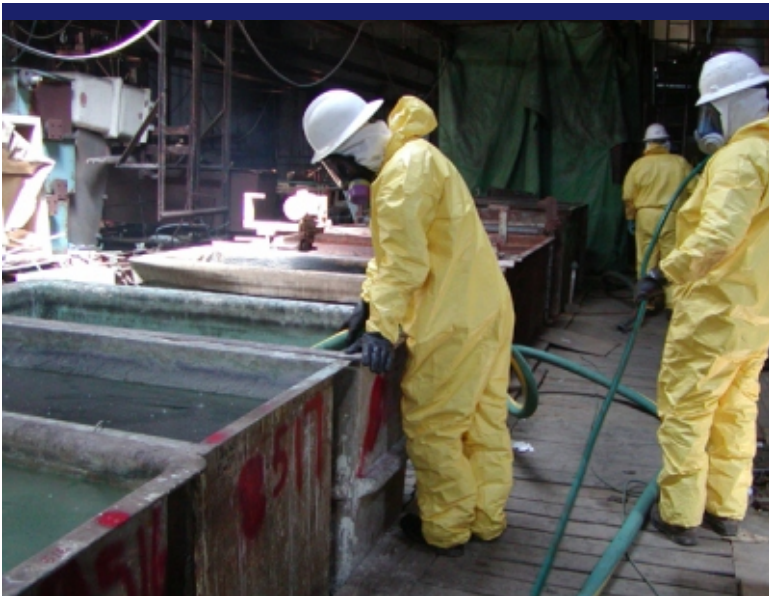
Photo 47 MPA: ERRS pumping out Plating Tank No. 518.
