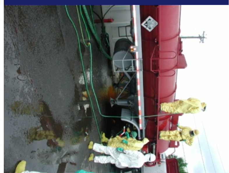
Photo 50 SSA: ERRS spraying down off-gas from PSC vacuum truck.
