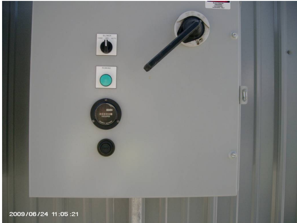
Aeration Picture 5 – Close up of Blower Pak Control Panel.
