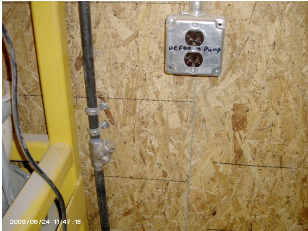
Defoamer Picture 5 – Dedicated timer controlled power receptacle for defoamer chemical feed pump. Timer control located in main control panel in 500k AST Pump House.
