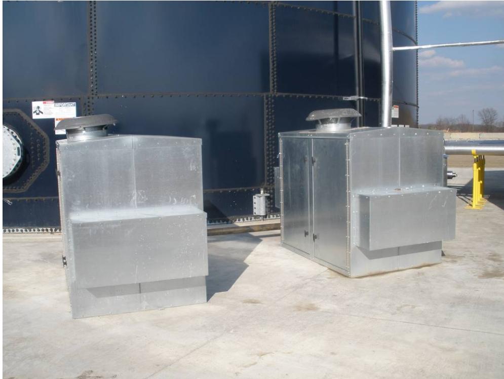
Aeration Picture 1 - Aeration Blower Packs at 500k AST-West.
