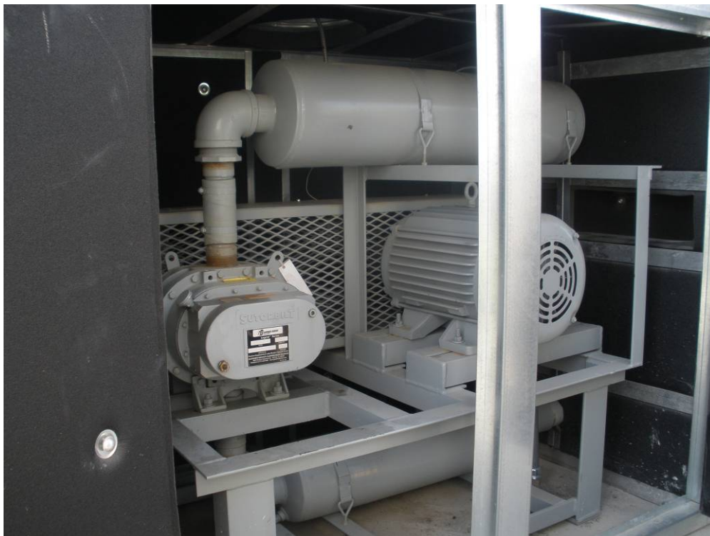
Aeration Picture 2 – Internal view 1 of Aeration Blower Pak.
