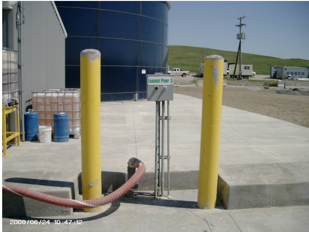
Loadout Picture 3 – 500k AST loadout station 3 of 3 and transfer hose. Operator's key switch located here.
