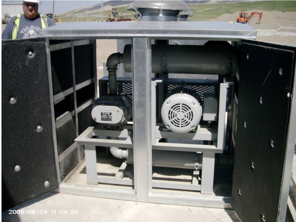
Aeration Picture 3 – Internal view 2 of Aeration Blower Pak.
