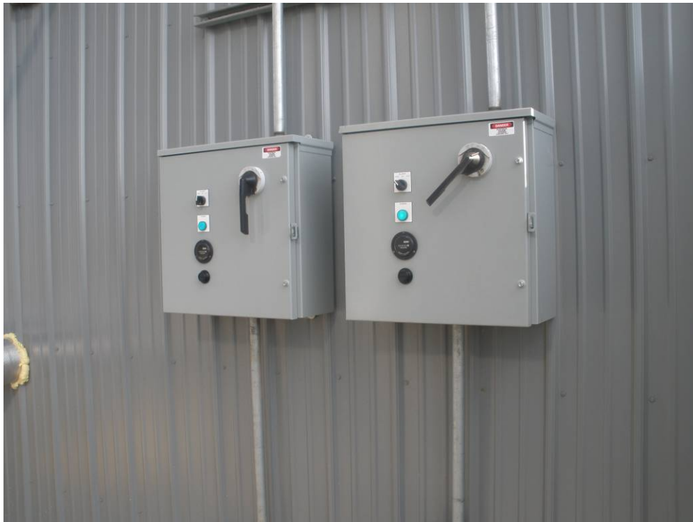
Aeration Picture 4 – Aeration Blower Pak control panels mounted on side of 500k AST Pump House. HOA switch control located here.
