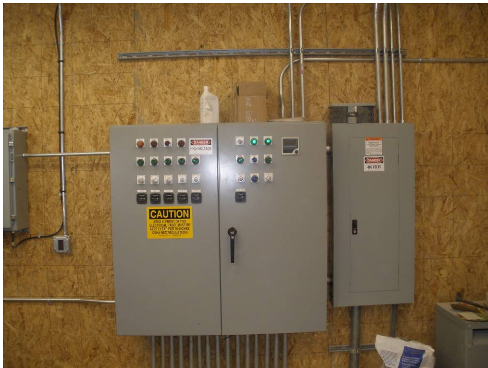
Aeration Picture 6 – Main control panel inside 500k AST Pump House. Thermatic Temperature Controller located here.
