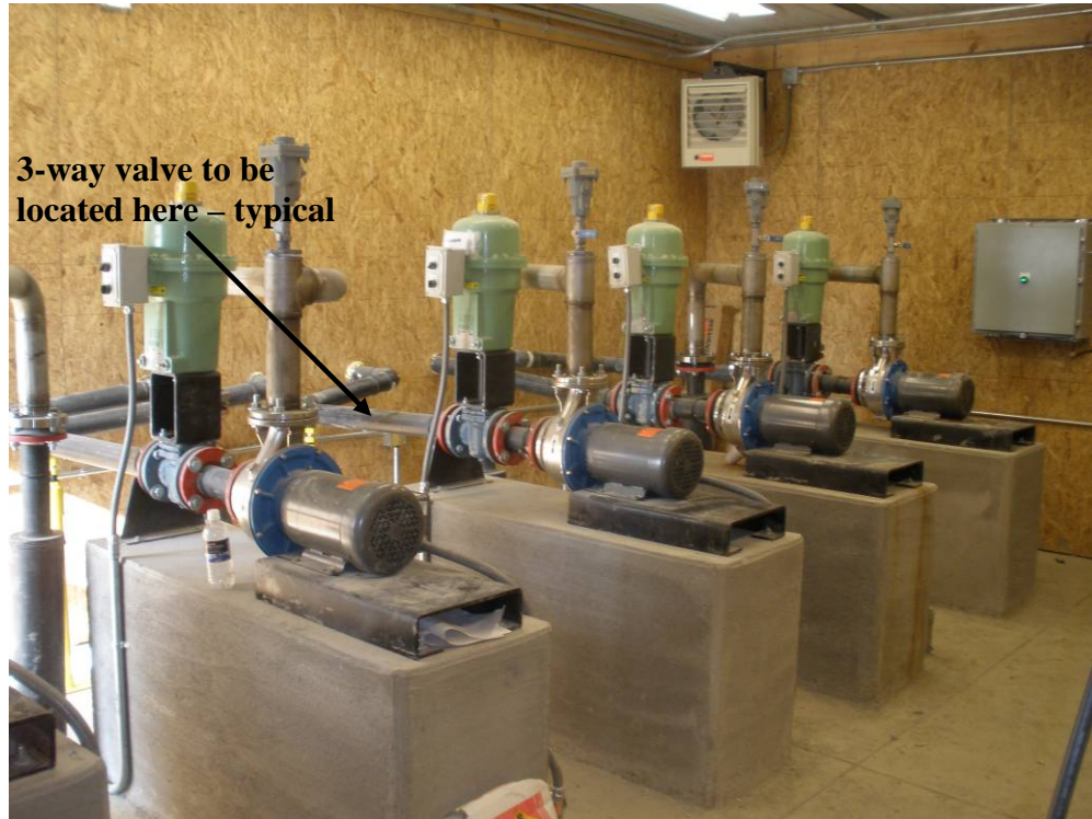
Loadout Picture 7 – 500k AST Transfer Pumps. Three-way valves used to select flow from 500k AST-West or 500k AST-East will be located here.
