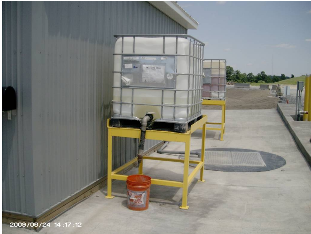
Defoamer Picture 1 – Mitfloc 5506L defoaming agent and transfer bucket. This station is moved inside the 500k AST Pump House during winter.
