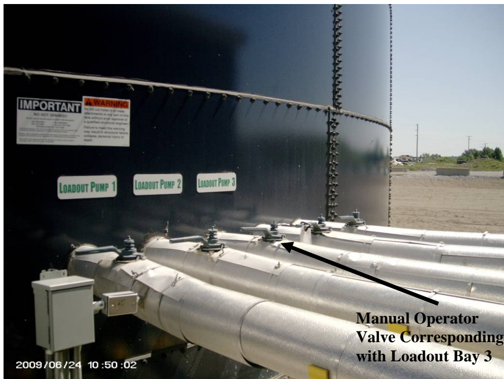
Loadout Picture 6 – Location of Manual Operator Valve. Open to allow flow to loadout pump corresponding with occupied loadout bay.
