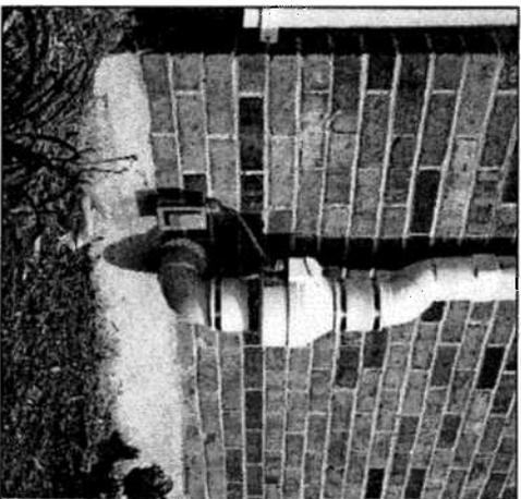
**Radon reduction system:** This system draws radon and other vapors out of the soil and vents them outside.
