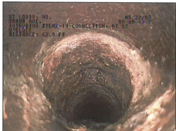
IMAGE: 150a, TAPE #: EMA-1, 02:07:31 62.9FT, intruding break-in-connection, at 02 o'clock
