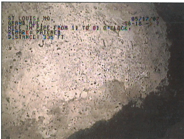
IMAGE: 84a, TAPE #: EMA-1, 01:17:21 335FT, Hole in pipe from 11 to 01 o'clock, REMARK: PATCHED
