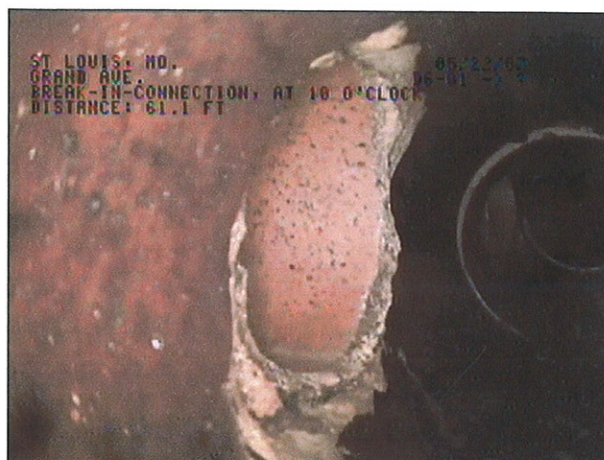
IMAGE: 167b, TAPE #: EMA-1, 02:14:03 61.1FT, break-in-connection, at 10 o'clock
