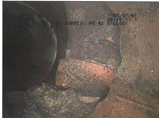
IMAGE: 83b, TAPE #: EMA-1, 01:16:51 333.8FT, service connection capped, at 02 o'clock
