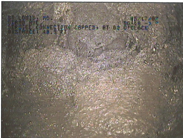
IMAGE: 51a, TAPE #: EMA-1, 01:00:26 40.9FT, service connection capped, at 03 o'clock
