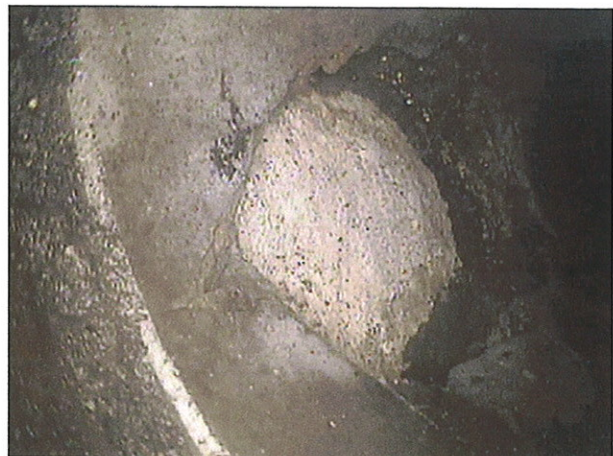
IMAGE: 84b, TAPE #: EMA-1, 01:17:21 335FT, Hole in pipe from 11 to 01 o'clock, REMARK: PATCHED
