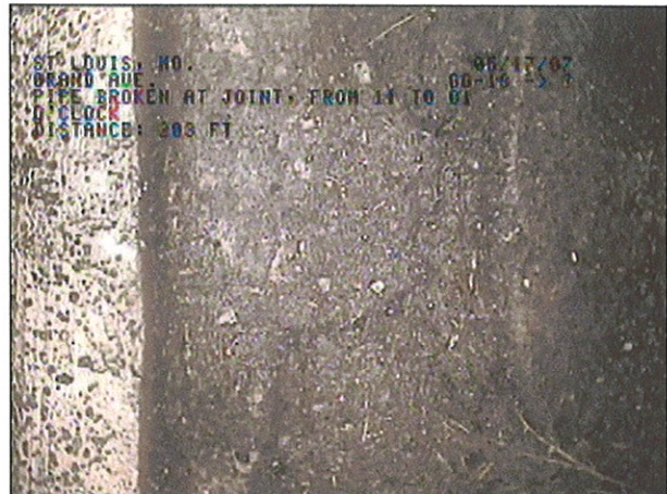
IMAGE: 69a, TAPE #: EMA-1, 01:09:36 203FT, pipe broken at joint, from 11 to 01 o'clock
