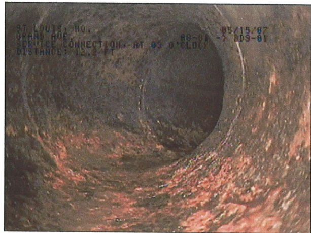
IMAGE: 33a, TAPE #: EMA-1, 00:40:04 12.2FT, service connection, at 03 o'clock
