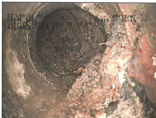
IMAGE: 102a, TAPE #: EMA-1, 01:28:30 17.5FT, service connection, at 10 o'clock
