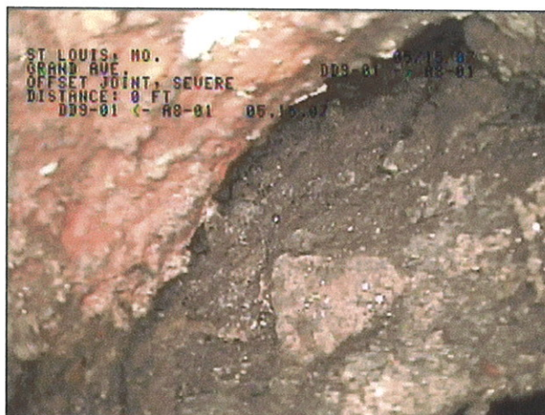
IMAGE: 30a, TAPE #: EMA-1, 00:36:12 2.5FT, offset joint, severe
