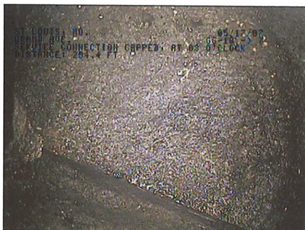
IMAGE: 76a, TAPE #: EMA-1, 01:12:39 254.4FT, service connection capped, at 03 o'clock
