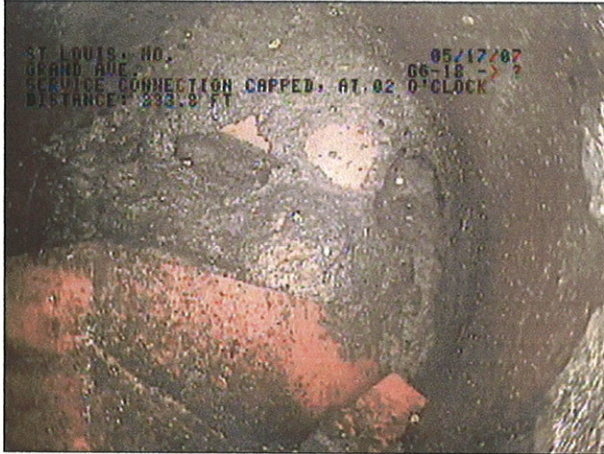
IMAGE: 83a, TAPE #: EMA-1, 01:16:51 333.8FT, service connection capped, at 02 o'clock
