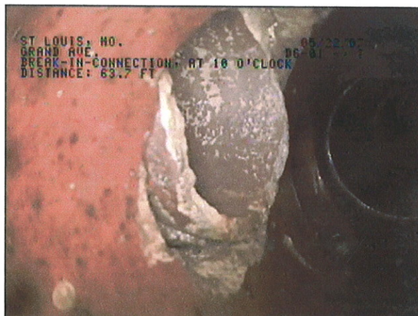
IMAGE: 168b, TAPE #: EMA-1, 02:14:26 63.7FT, break-in-connection, at 10 o'clock
