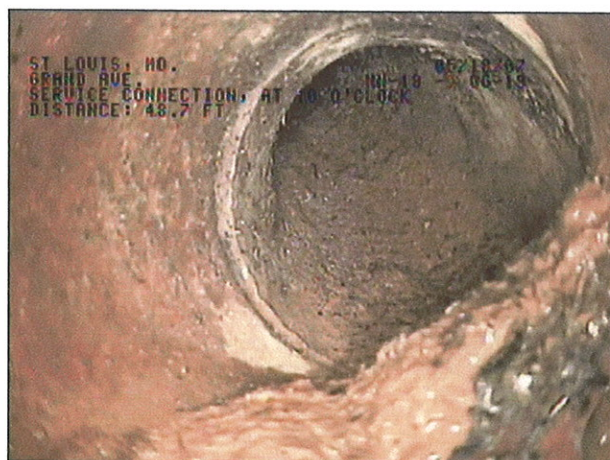
IMAGE: 103a, TAPE #: EMA-1, 01:29:16 48.7FT, service connection, at 10 o'clock
