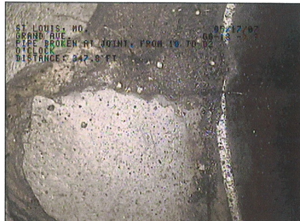
IMAGE: 86a, TAPE #: EMA-1, 01:18:19 347.8FT, pipe broken at joint, from 10 to 02 o'clock
