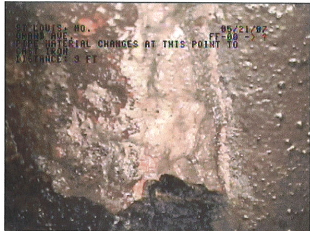
IMAGE: 141a, TAPE #: EMA-1, 02:01:36 9FT, pipe material changes at this point to cast iron
