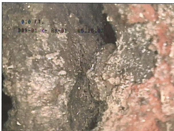
IMAGE: 30b, TAPE #: EMA-1, 00:36:12 2.5FT, offset joint, severe
