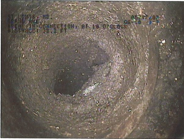
IMAGE: 50a, TAPE #: EMA-1, 00:59:53 38.3FT, break-in-connection, at 10 o'clock
