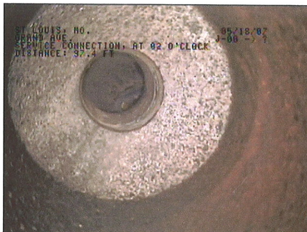
IMAGE: 129a, TAPE #: EMA-1, 01:48:12 97.4FT, service connection, at 02 o'clock
