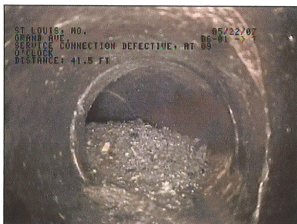
IMAGE: 164a, TAPE #: EMA-1, 02:13:00 41.5FT, service connection defective, at 09 o'clock
