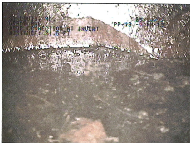
IMAGE: 112a, TAPE #: EMA-1, 01:36:28 21.5FT, drop connection at invert
