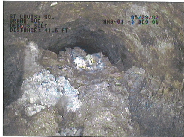
IMAGE: 187a, TAPE #: EMA-1, 02:29:35 41.5FT, debris silt
