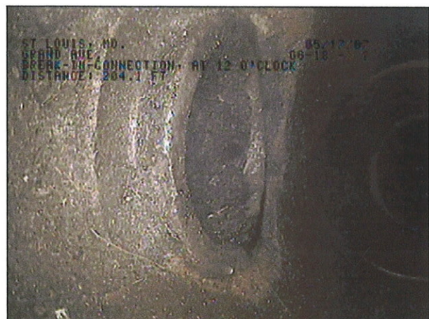
IMAGE: 70b, TAPE #: EMA-1, 01:09:49 204.1FT, break-in-connection, at 12 o'clock
