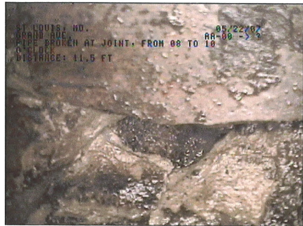
IMAGE: 146a, TAPE #: EMA-1, 02:05:11 11.5FT, pipe broken at joint, from 08 to 10 o'clock
