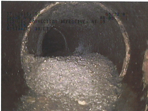
IMAGE: 149a, TAPE #: EMA-1, 02:06:38 39FT, service connection defective, at 09 o'clock
