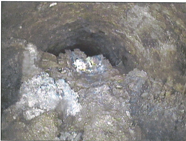
IMAGE: 188a, TAPE #: EMA-1, 02:29:42 41.5FT, camera blocked, inspection abandoned
