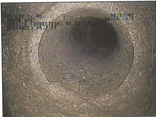
IMAGE: 55a, TAPE #: EMA-1, 01:02:26 85.2FT, service connection, at 02 o'clock
