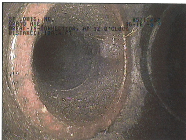
IMAGE: 59b, TAPE #: EMA-1, 01:04:37 120.4FT, break-in-connection, at 12 o'clock
