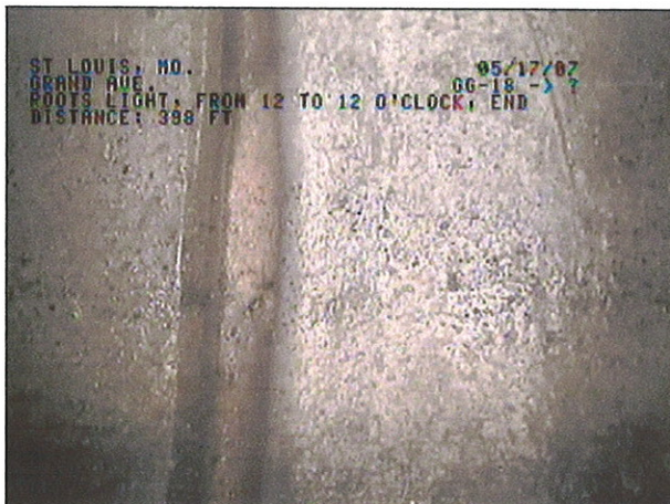
IMAGE: 91a, TAPE #: EMA-1, 01:20:57 398FT, roots light, from 12 to 12 o'clock, END
