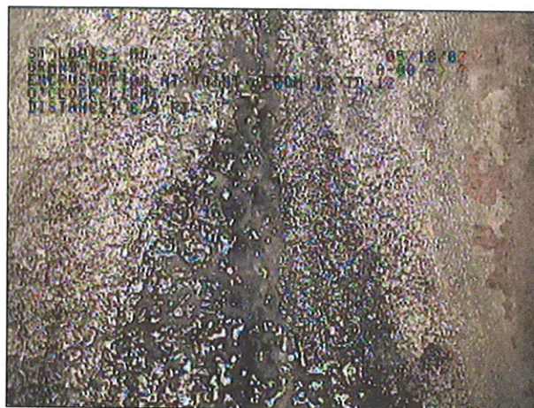
IMAGE: 132a, TAPE #: EMA-1, 01:52:53 6.8FT, encrustation at joint, from 12 to 12 o'clock light, START
