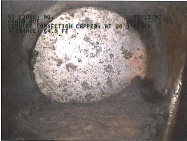
IMAGE: 169a, TAPE #: EMA-1, 02:14:44 64.5FT, service connection capped, at 10 o'clock
