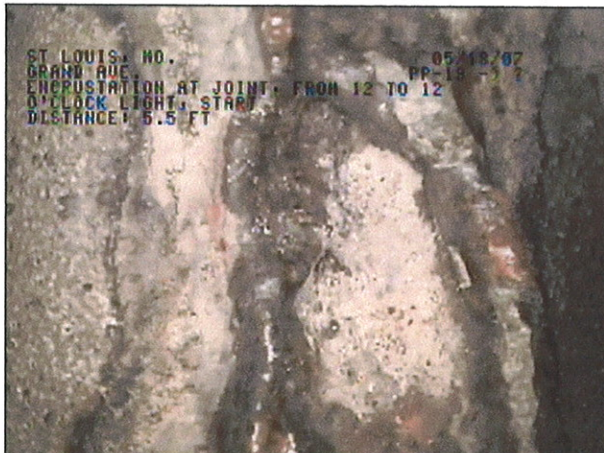
IMAGE: 116a, TAPE #: EMA-1, 01:39:12 5.5FT, encrustation at joint, from 12 to 12 o'clock light, START
