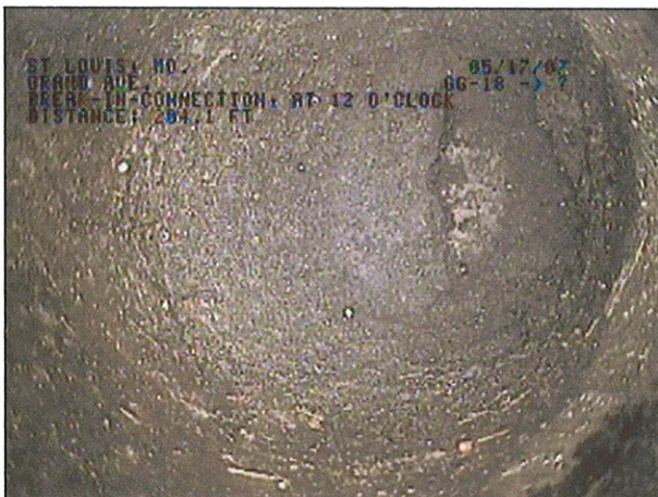
IMAGE: 70a, TAPE #: EMA-1, 01:09:49 204.1FT, break-in-connection, at 12 o'clock
