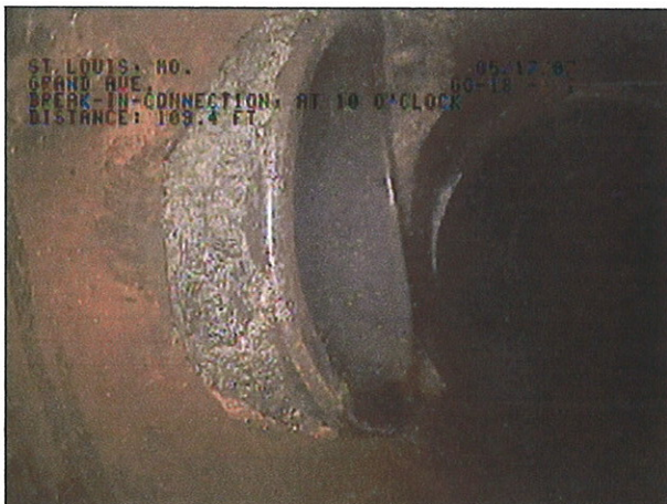
IMAGE: 58b, TAPE #: EMA-1, 01:03:44 109.4FT, break-in-connection, at 10 o'clock
