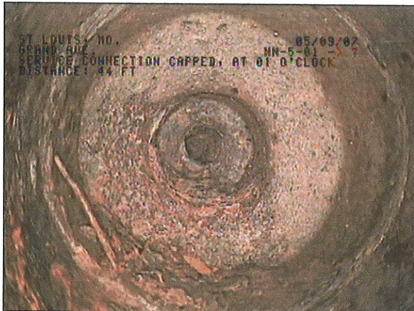
IMAGE: 9a, TAPE #: EMA-1, 00:10:00 44FT, service connection capped, at 01 o'clock
