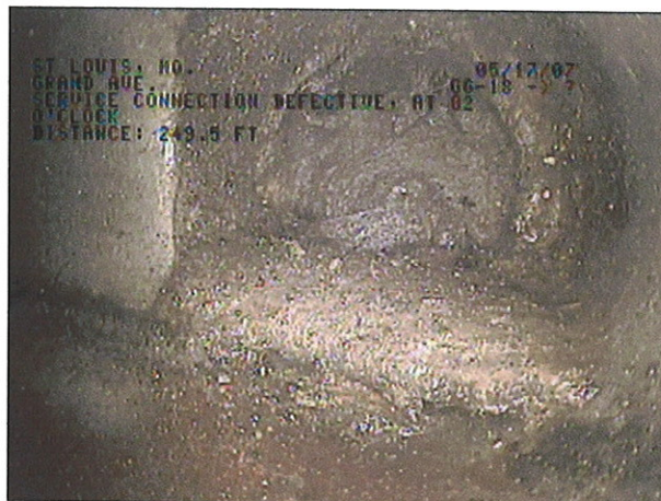
IMAGE: 75a, TAPE #: EMA-1, 01:12:15 249.4FT, service connection defective, at 02 o'clock
