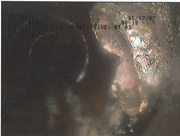
IMAGE: 48b, TAPE #: EMA-1, 00:58:36 17FT, break-in-connection defective, at 03 o'clock
