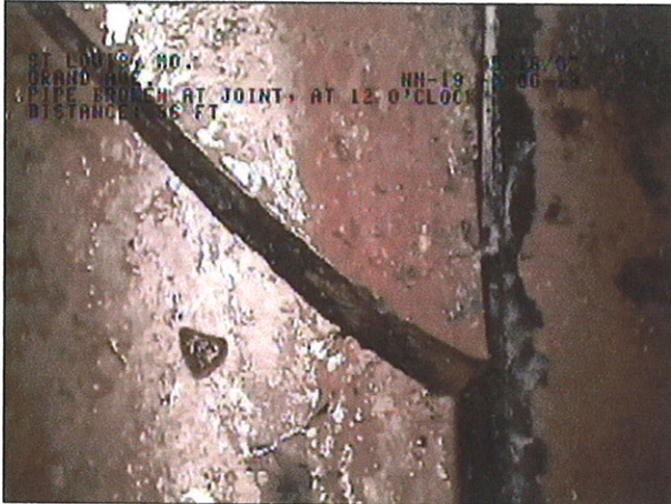
IMAGE: 105a, TAPE #: EMA-1, 01:30:33 96FT, pipe broken at joint, from 10 to 11 o'clock
