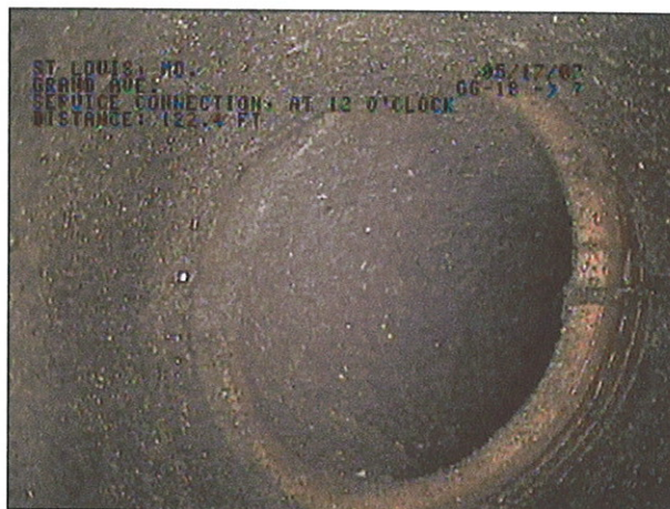
IMAGE: 60a, TAPE #: EMA-1, 01:05:07 122.4FT, service connection, at 12 o'clock
