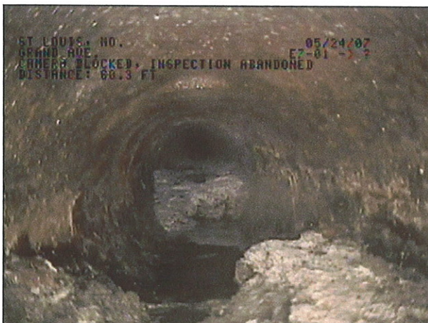
IMAGE: 181a, TAPE #: EMA-1, 02:22:29 60.3FT, camera blocked, inspection abandoned
