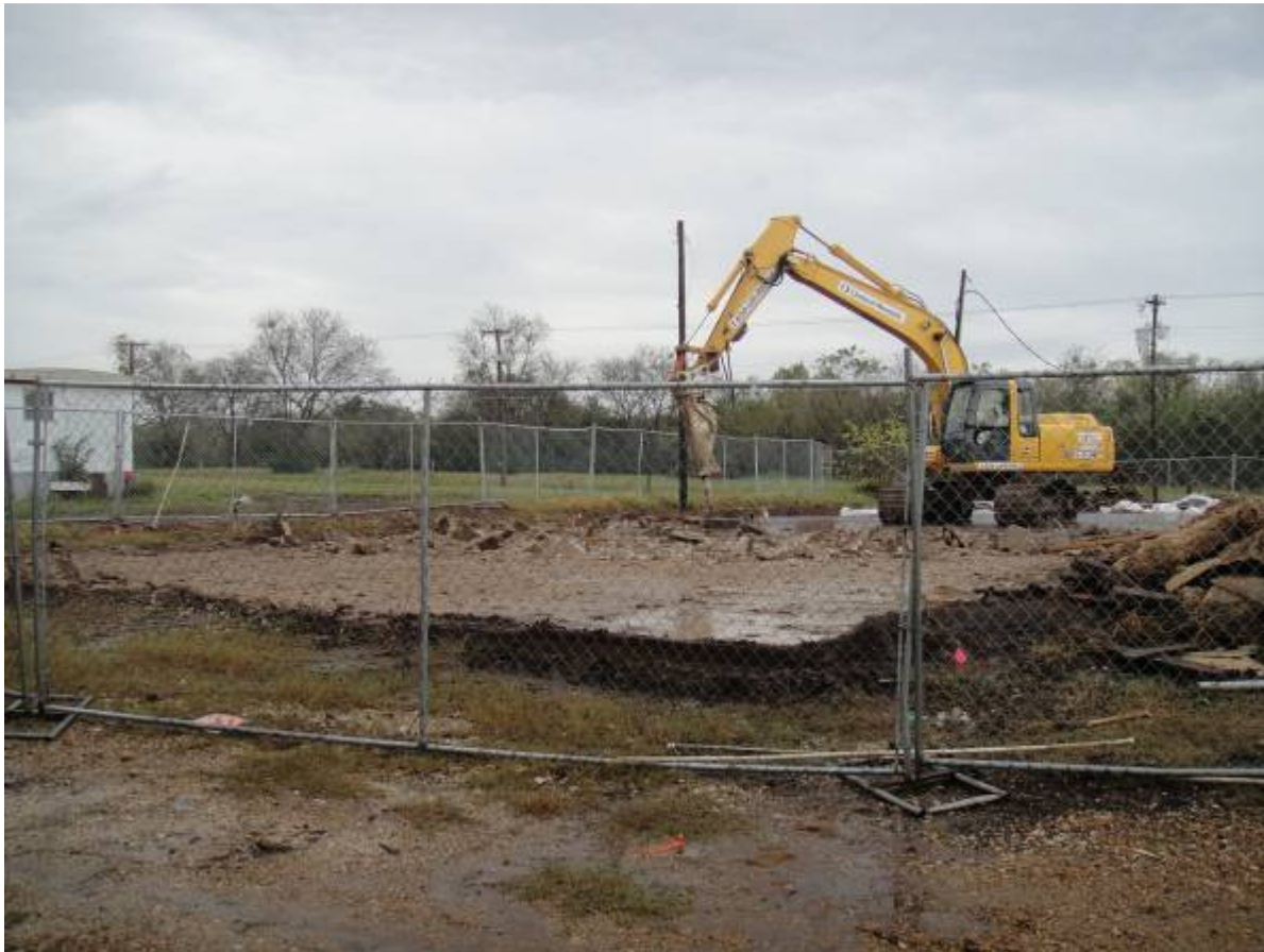
Breaking up concrete pad
