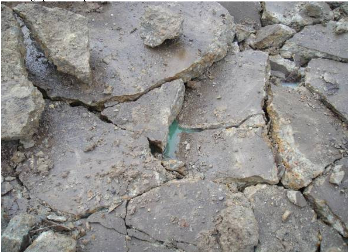
Discolored liquid under concrete pad
