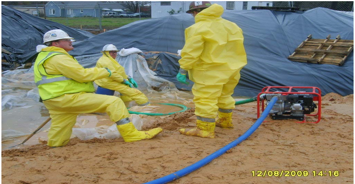
View of ERRS pumping pooled rain water from excavation (JPG S5000524).
