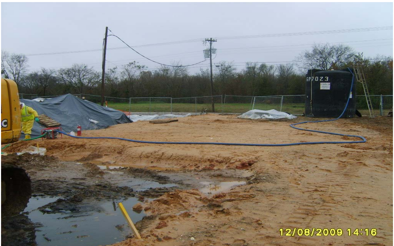
View of ERRS pumping pooled rain water from excavation and into 6,500 gallon poly AST. (JPGS5000525).
