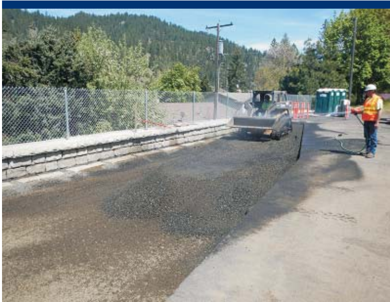
Photo 69 Placement of final lift in asphalt repair area.
