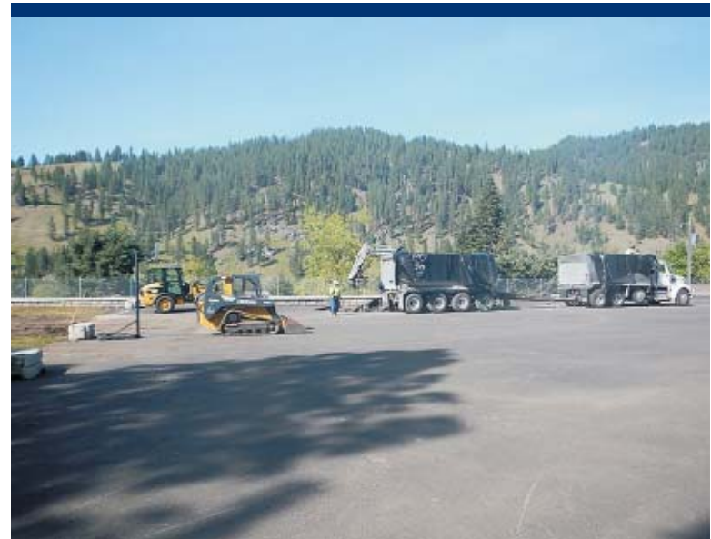
Photo 24 Loading waste into lined truck and pup.
