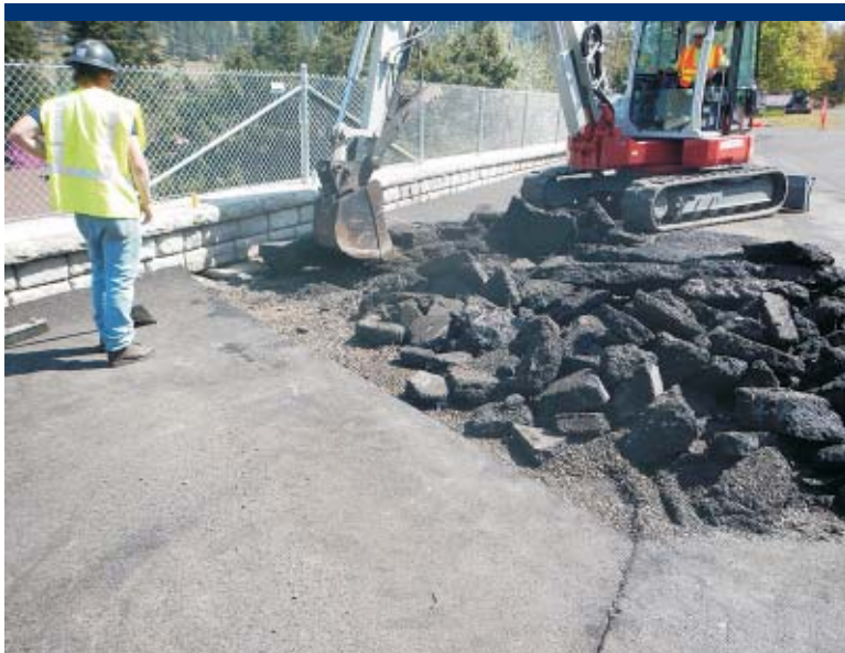
Photo 7 ERRS removes asphalt from asphalt repair area.
