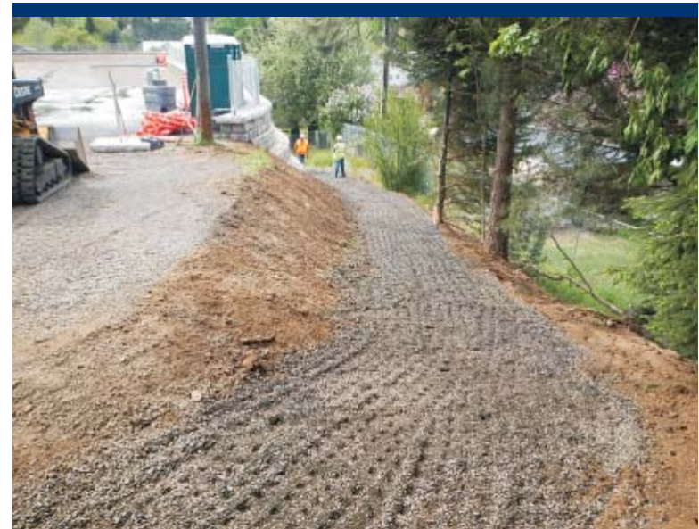
Photo 88 Final lower access ramp and gravel, compacted.
