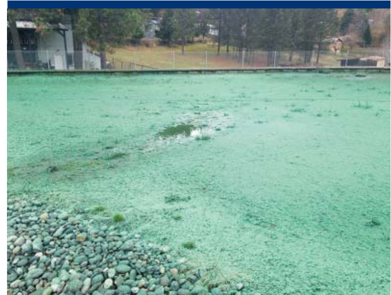
Photo 112 Dry retention basin with hydroseed and mulch applied.
