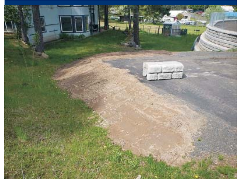
Photo 58 Ramp to decrease dropoff angle at southwest corner of asphalt cap.
