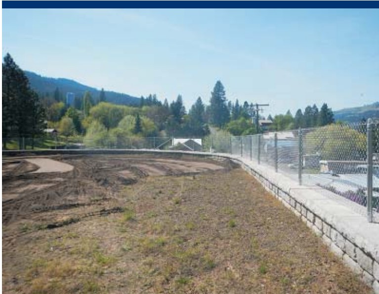
Photo 17 Top soil is spread on a portion of the dry retention basin.
