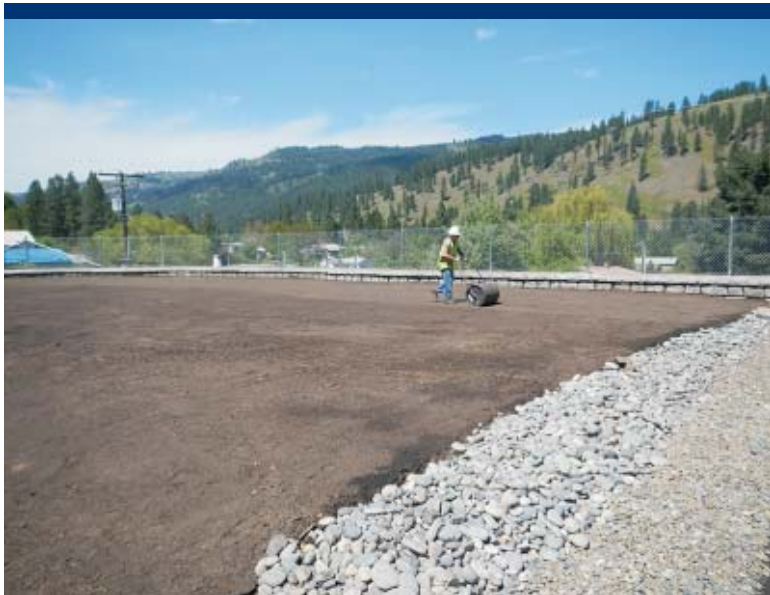
Photo 84 Rolling seed into dry retention basin with water barrel roller.
