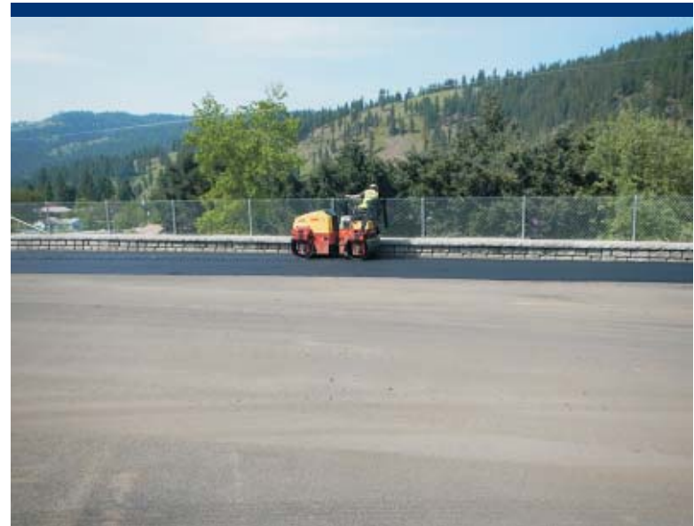
Photo 96 Compacting first lift of asphalt repair patch.
