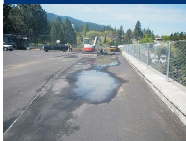
Photo 6 View of excavator breaking asphalt, and puddled water in asphalt repair area.
