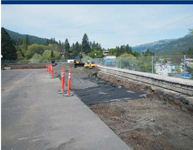
Photo 37 Backfill of asphalt repair area with 3/4-inch minus aggregate on geotextile.
