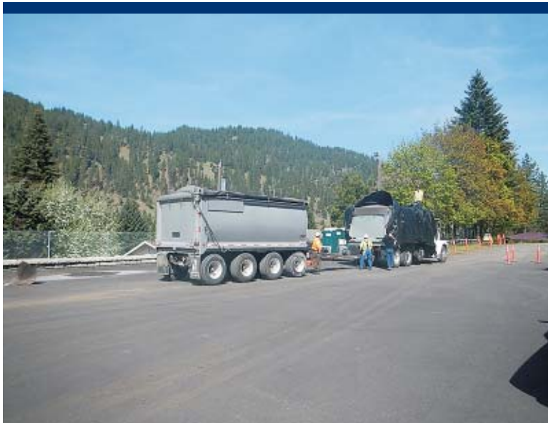
Photo 19 ERRS lines the back of an off-site haul truck.
