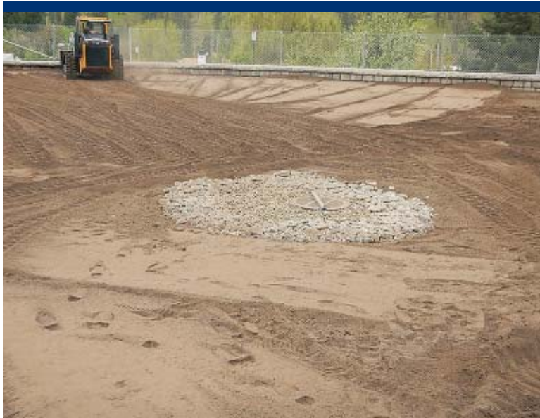
Photo 49 Completed dry well/CMP upgrade.
