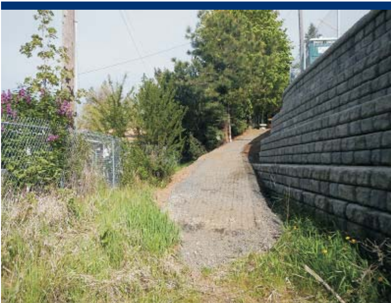
Photo 87 Final lower access ramp and gravel, compacted.
