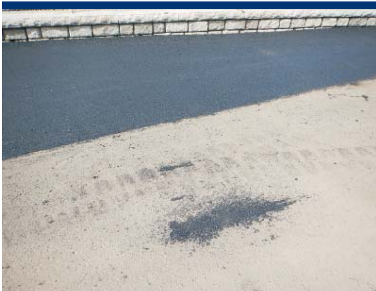
Photo 99 Repaired gouge in asphalt patched by paving contractor.
