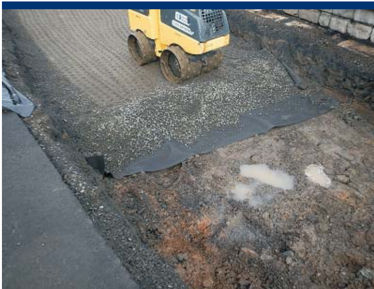
Photo 51 Edge of backfill lift with compactor.
