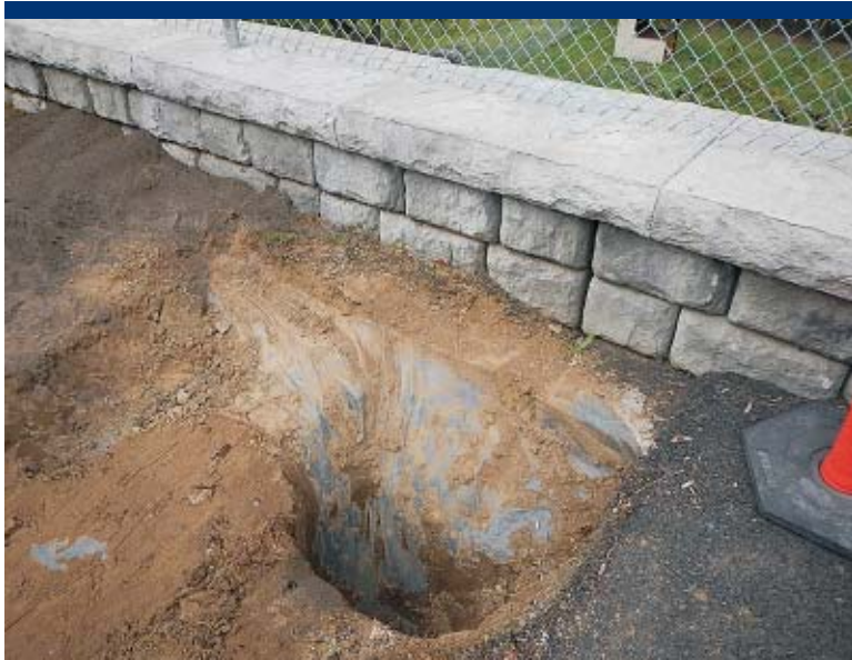
Photo 45 PVC liner and anchor trench of dry retention basin.
