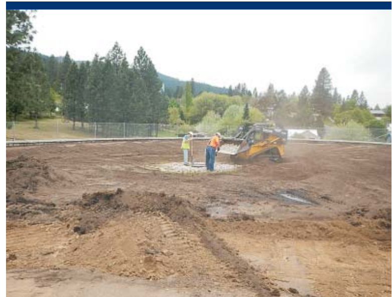
Photo 48 ERRS installs washed rock around dry well.
