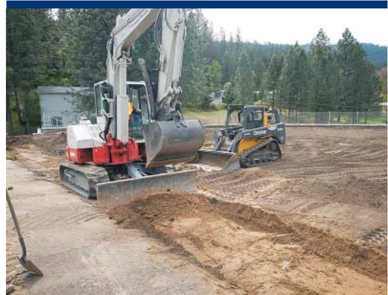
Photo 46 Excavating at drain rock apron.
