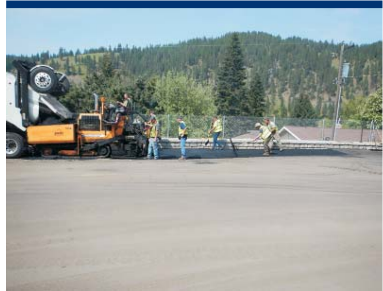
Photo 94 Placement of first asphalt lift.
