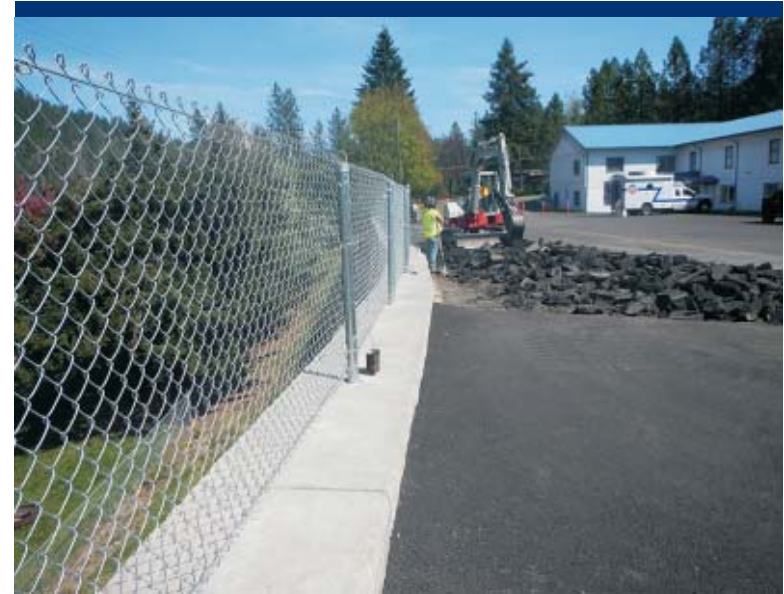
Photo 14 ERRS removes asphalt from asphalt repair area; air sampling pump in foreground.
