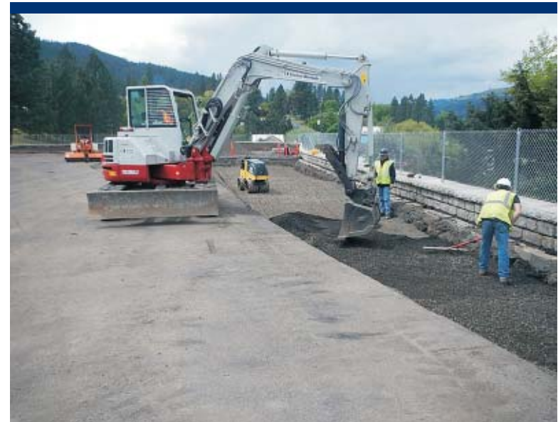
Photo 64 Backfilling asphalt repair area, placing in 6-inch lifts.
