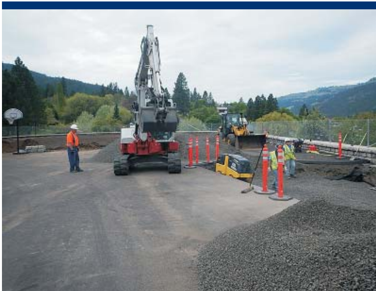
Photo 43 Backfill and compaction.
