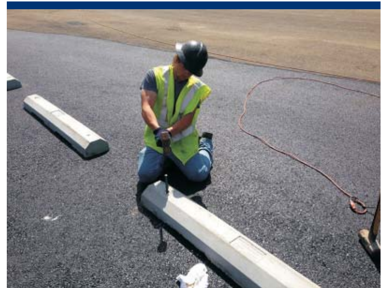
Photo 104 Installation of parking space stopper.
