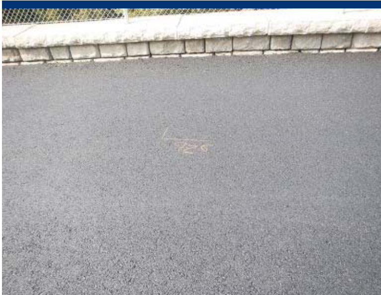
Photo 101 Compaction results for asphalt repair area.
