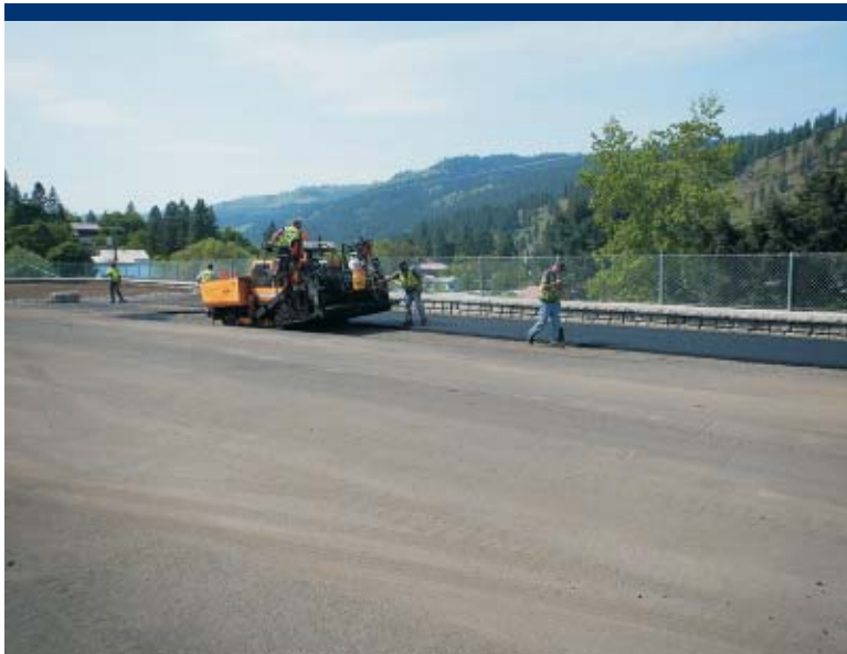
Photo 95 Placement of first asphalt lift.
