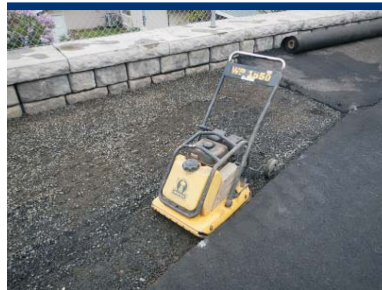
Photo 80 Mini compactor for final grade of backfill in asphalt repair area.
