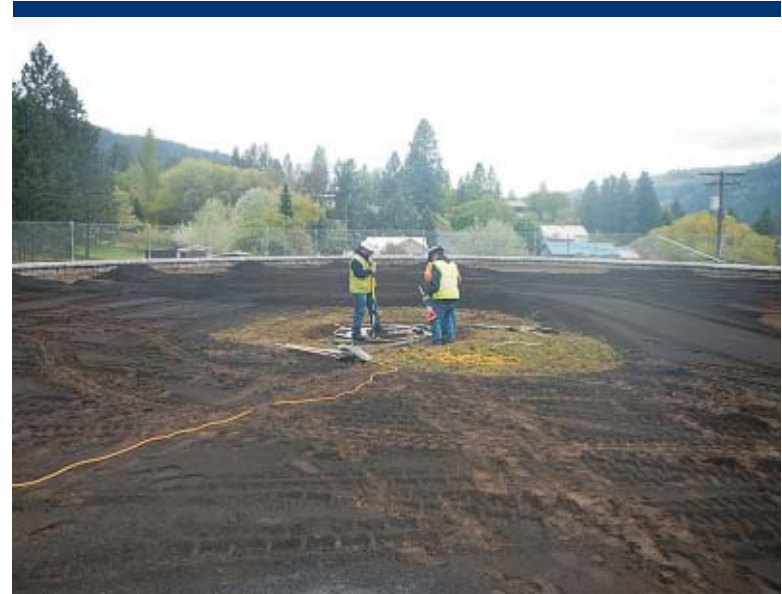
Photo 30 Work begins on corrugated metal pipe (CMP) around dry well.
