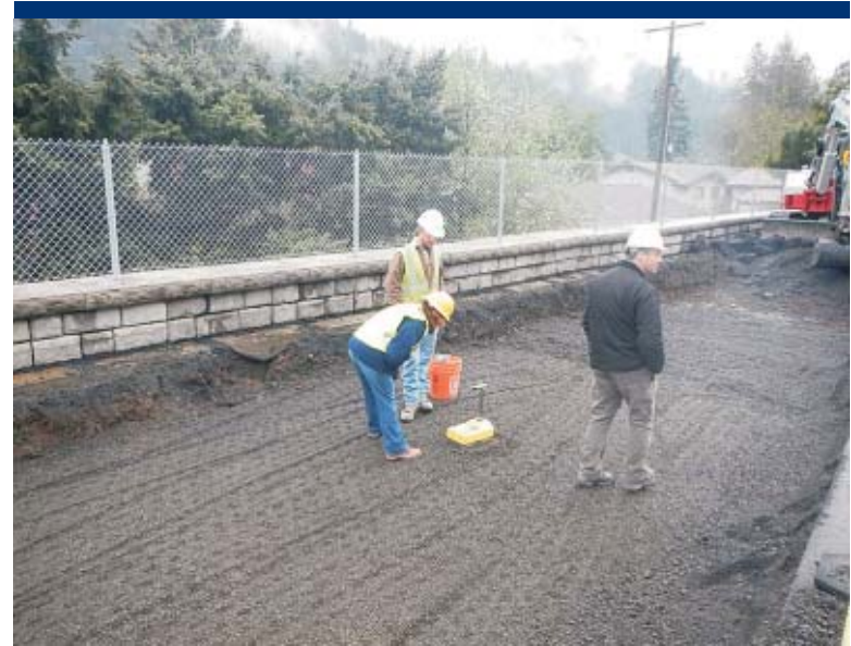
Photo 50 Compaction testing with OSC and ERRS RM.
