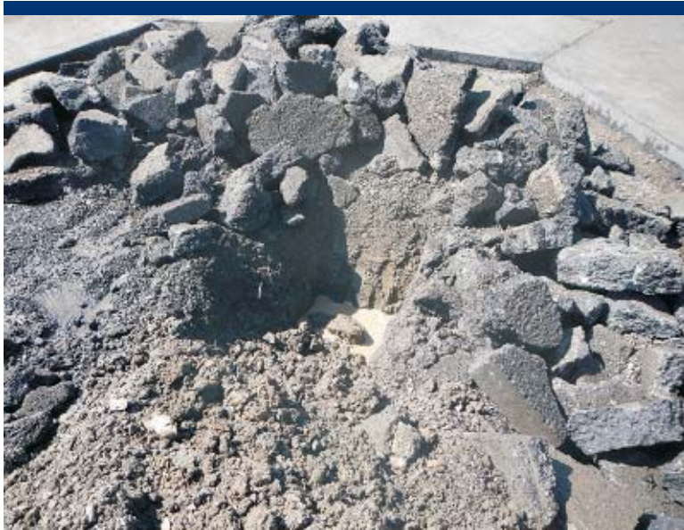
Photo 9 Water at interface of asphalt/sub-base and contaminated fill.
