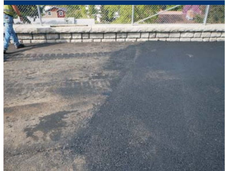
Photo 98 Photo shows small float coat of asphalt placed in low area of existing west asphalt patch.
