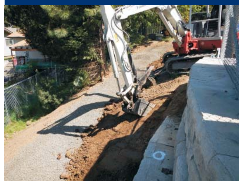
Photo 86 Bringing access ramp side slopes to grade.
