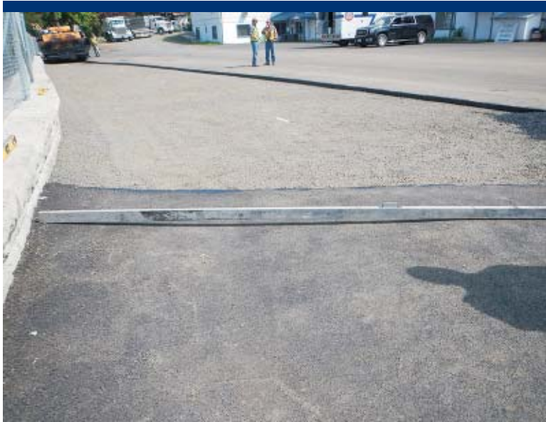
Photo 93 Straight edge showing settling of existing west asphalt repair.
