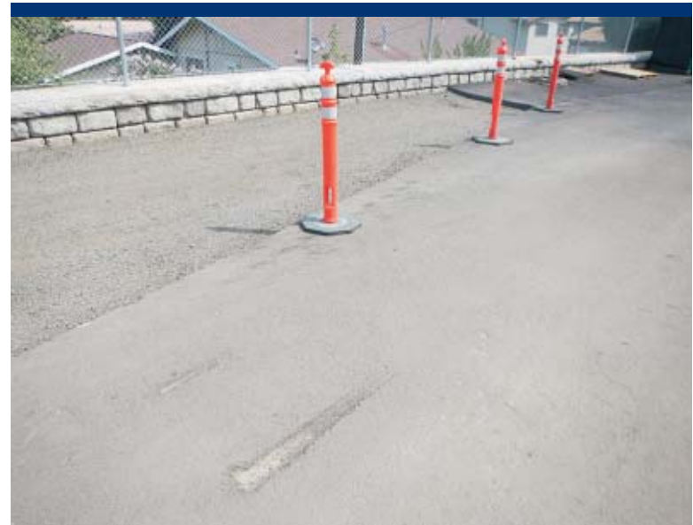
Photo 100 Gouge in asphalt to be patched by paving contractor.
