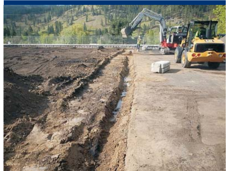
Photo 54 Excavation in drain rock apron area.
