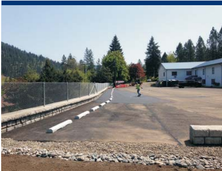
Photo 106 Overview of sealed asphalt repair area and installed parking space stoppers. Direction: East Date: 5/4/15 Time: 11:19 Taken by: ERRS
