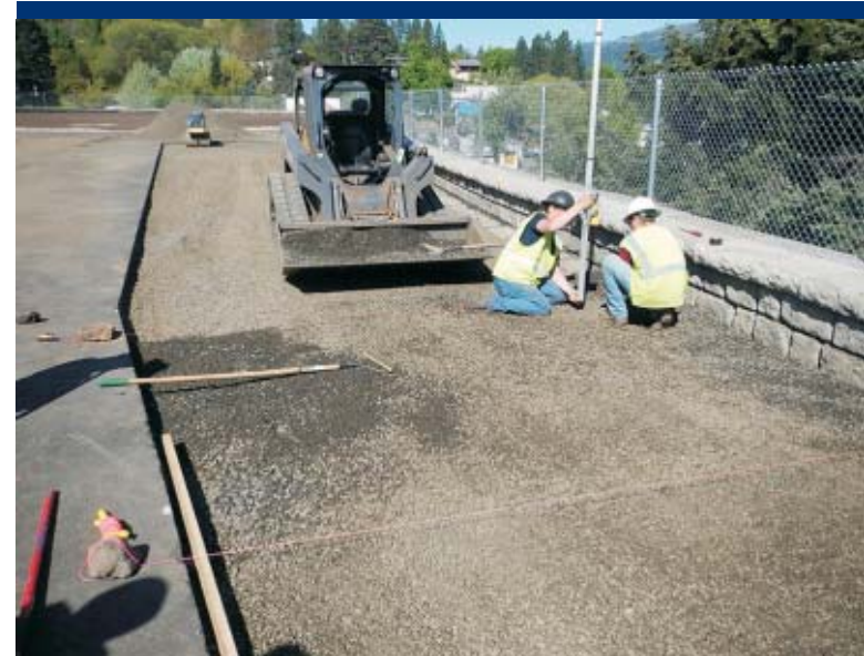
Photo 78 Surveying backfill elevation for final grade.
