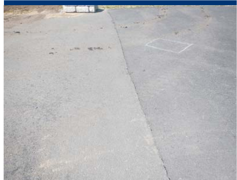
Photo 10 Seam from 2012 asphalt repair.
