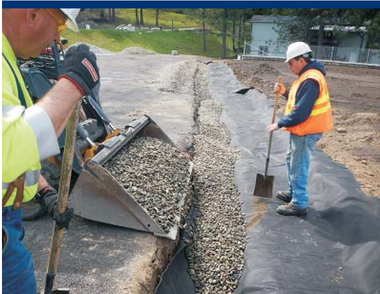
Photo 57 Placing drain rock in trench.
