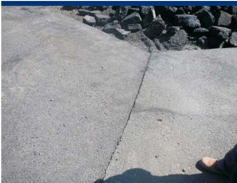
Photo 11 Seam from 2012 asphalt repair.
