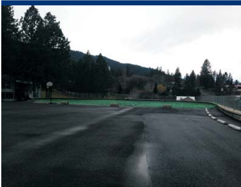
Photo 114 Overview of parking lot drainage and hydroseeded dry retention basin.
