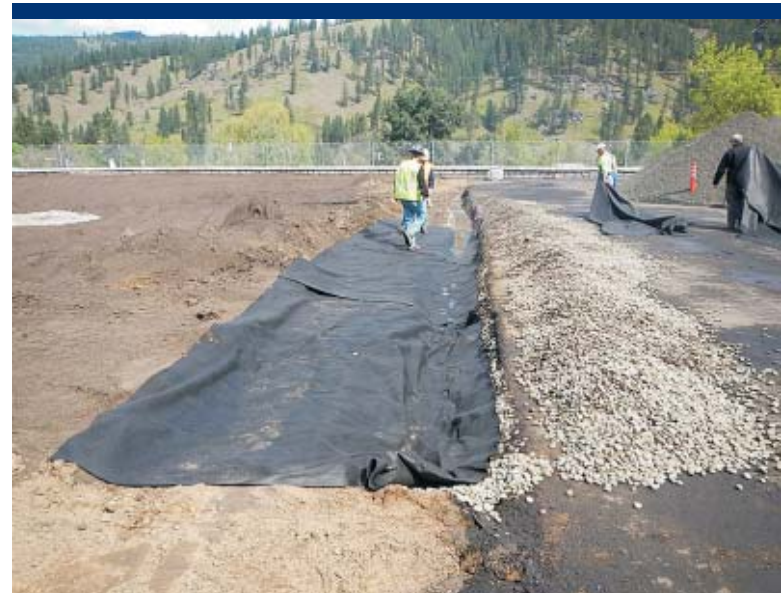
Photo 56 Placement of geotextile in drain rock apron.
