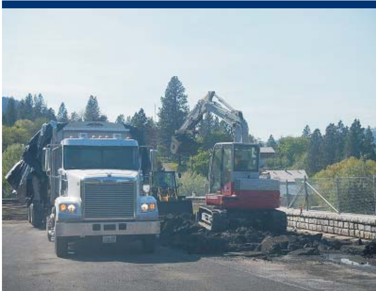
Photo 21 Loading waste into lined truck and pup.
