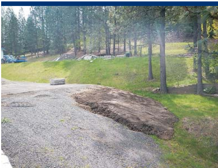
Photo 59 Ramp to decrease dropoff angle at southwest corner of asphalt cap.
