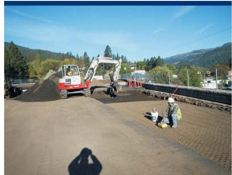
Photo 68 Placement of backfill lift, and compaction testing.
