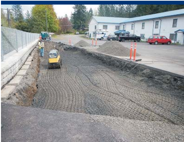
Photo 47 Compaction of aggregate.
