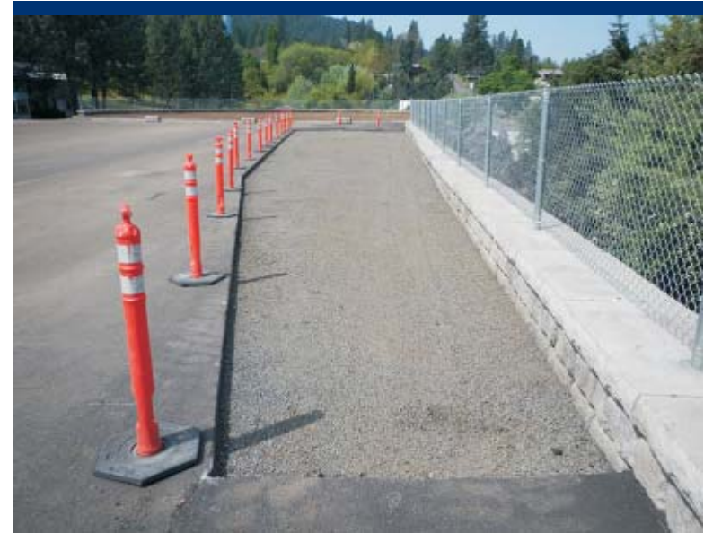
Photo 90 Asphalt repair area ready for paving.
