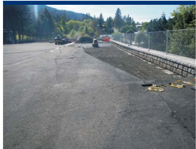
Photo 76 Backfilled asphalt repair area.
