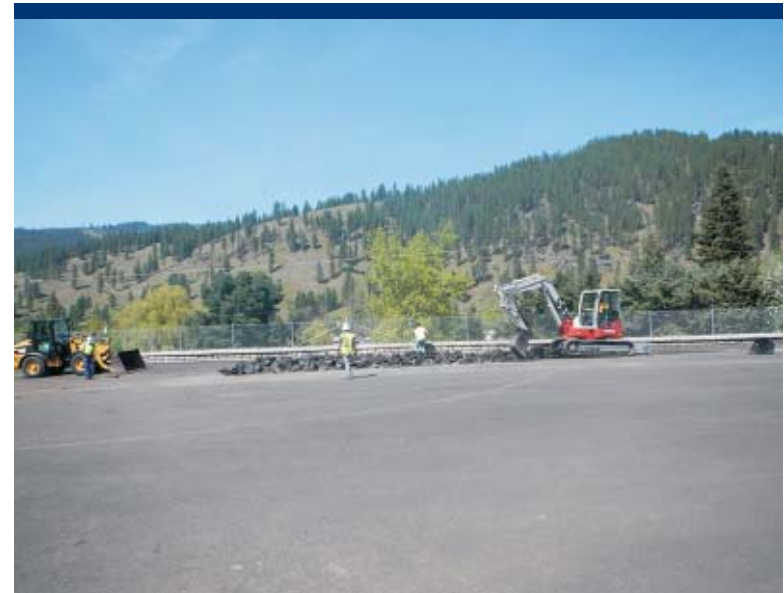
Photo 16 ERRS removes asphalt from asphalt repair area.
