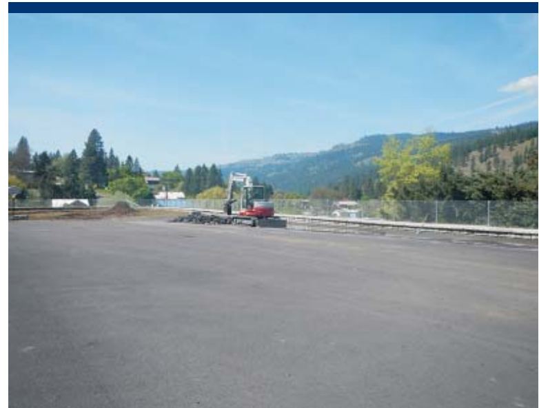
Photo 12 ERRS removing asphalt from asphalt repair area.
