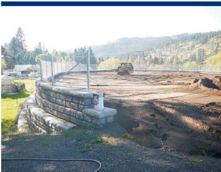
Photo 35 Spreading topsoil on dry retention basin; DataRAM #3 in foreground.
