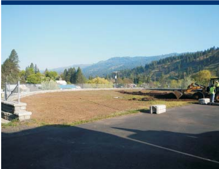
Photo 1 Placing top soil on dry retention basin.
