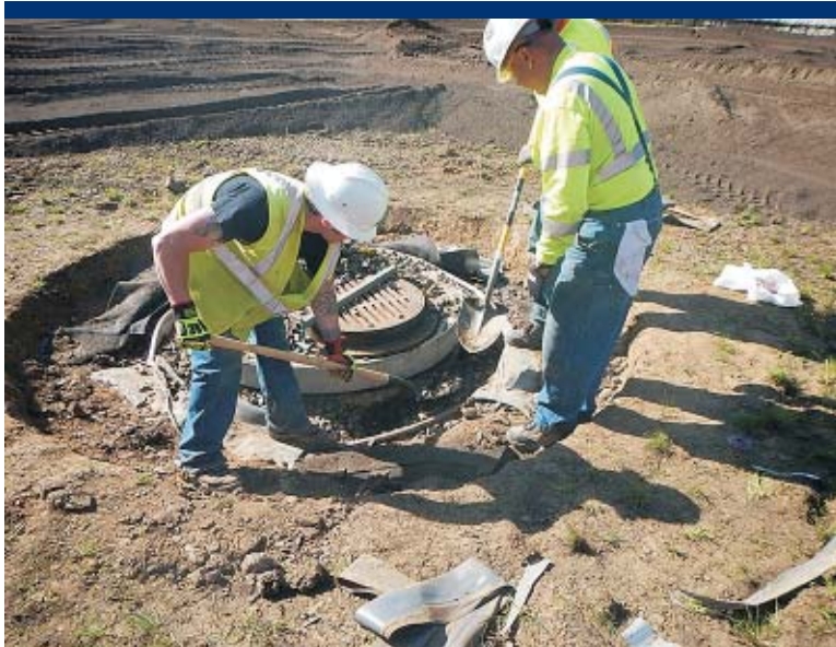
Photo 33 ERRS places PVC liner inside CMP.
