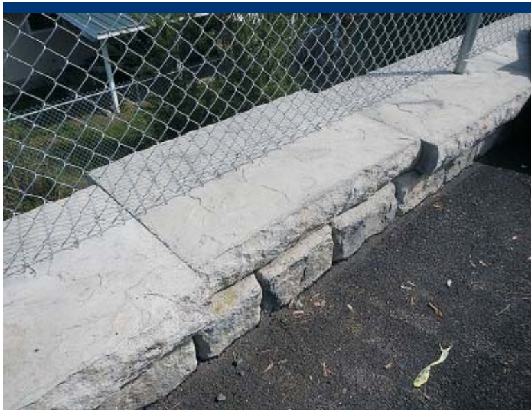
Photo 55 Displaced top cap along top of retaining wall.
