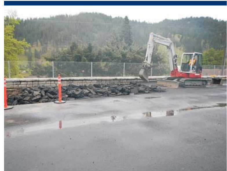
Photo 28 Removing asphalt from central asphalt repair area.
