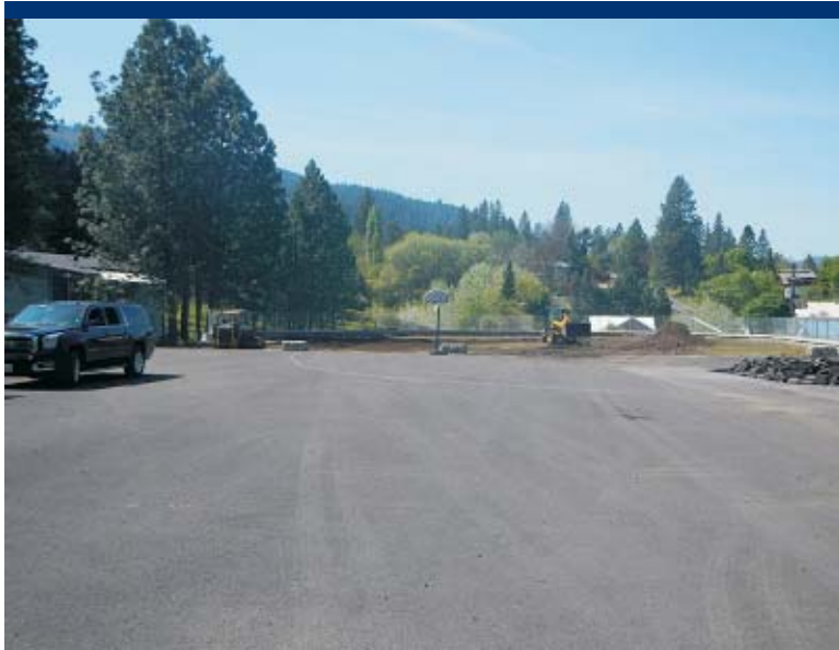
Photo 13 Spreading topsoil on dry retention basin.
