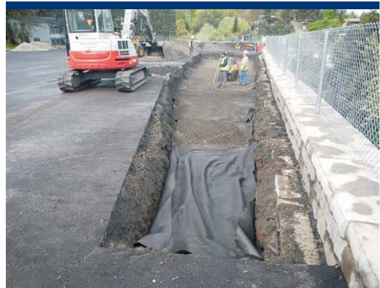
Photo 52 Backfilling asphalt repair area.
