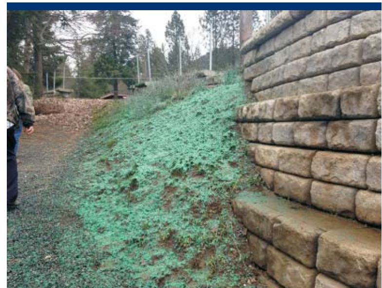
Photo 113 Hydroseed and mulch applied to slope on uphill side of northeast access ramp.
