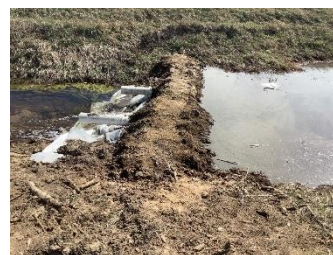
Earthen berm and underflow dam in the ditch that runs west of I-25. Underflow dam has been reinforced and boom removed.
