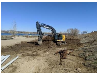
Primary area of contaminated soil excavation west of I-25 South. Area was heavily saturated with diesel product and main collection point during initial response actions.
