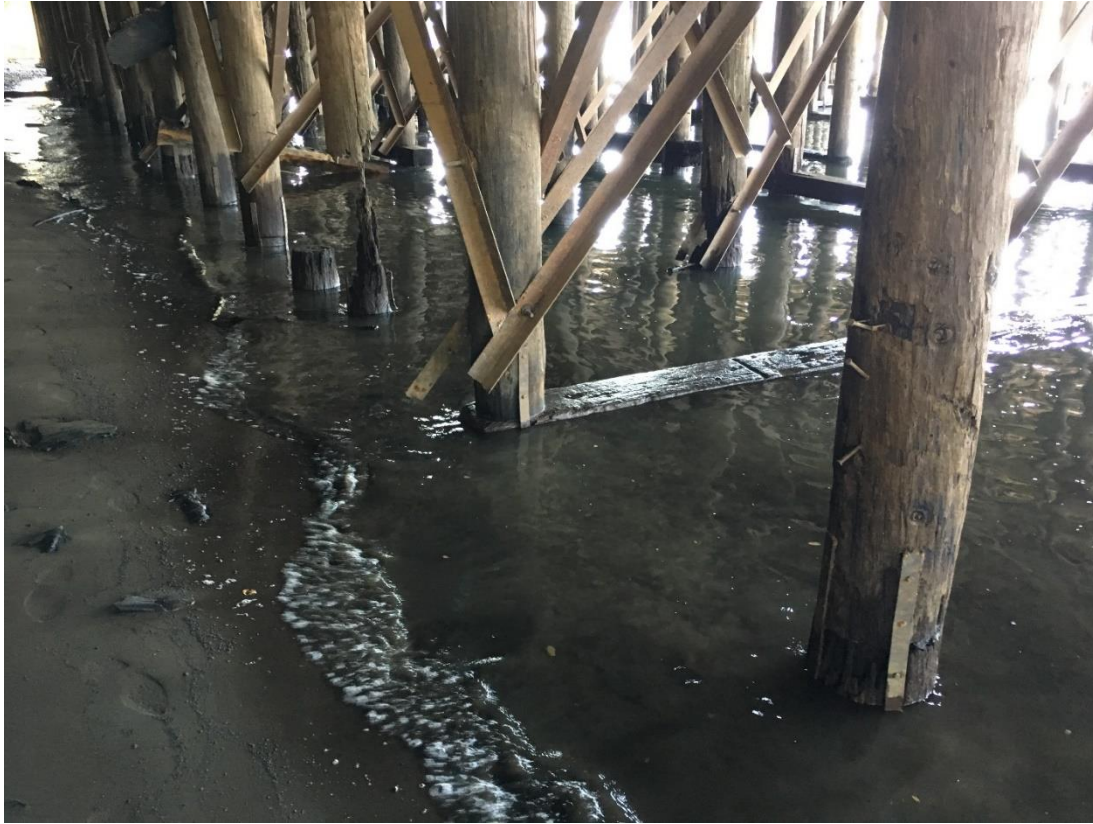
Photo #7 – Pile bent at waterline with straps exposed to indicate piles have been spliced. Note rotted pile in upper right area of photo.
