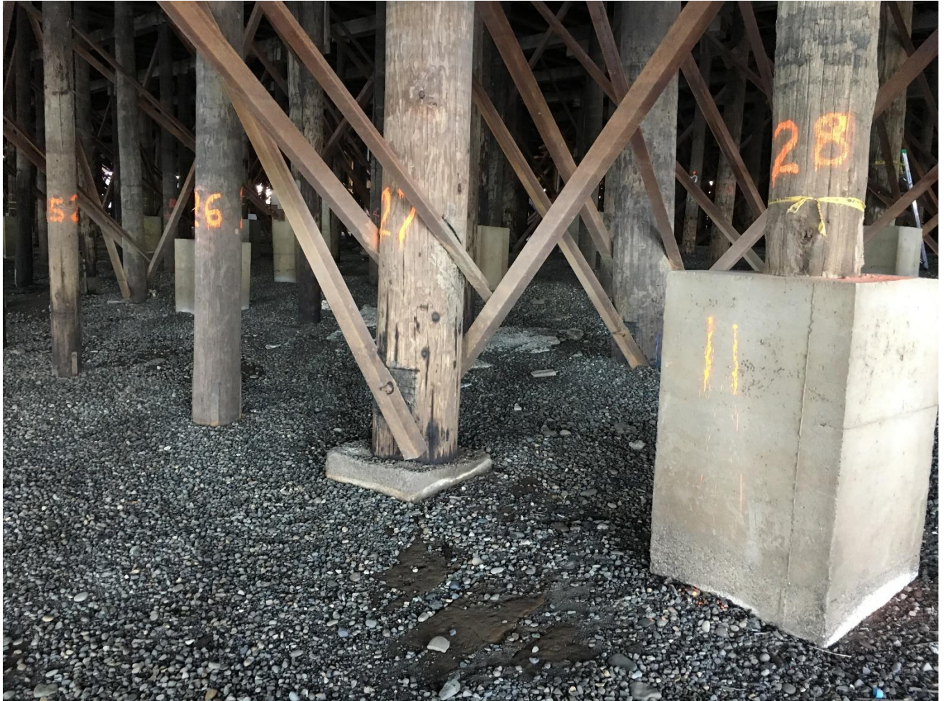
Photo #6 – Typical pile bent on shore with pile splice hidden below ground, but straps indicate that the pile has been spliced. It is assumed that the concrete blocks shown in this photo encase pile splice joints.
