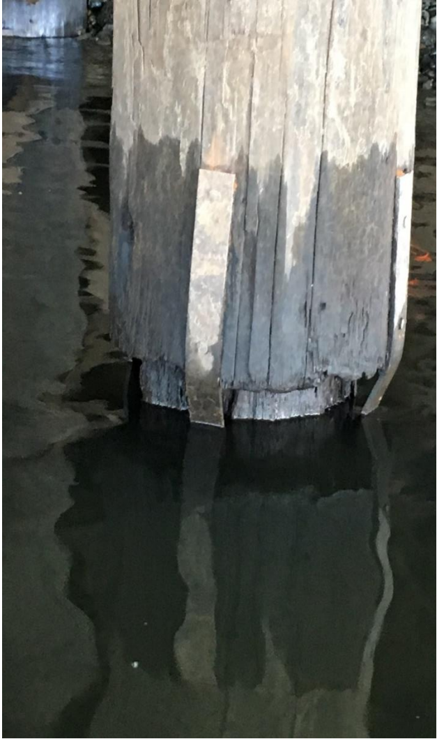
Photo #2 – Typical pile splice at waterline
