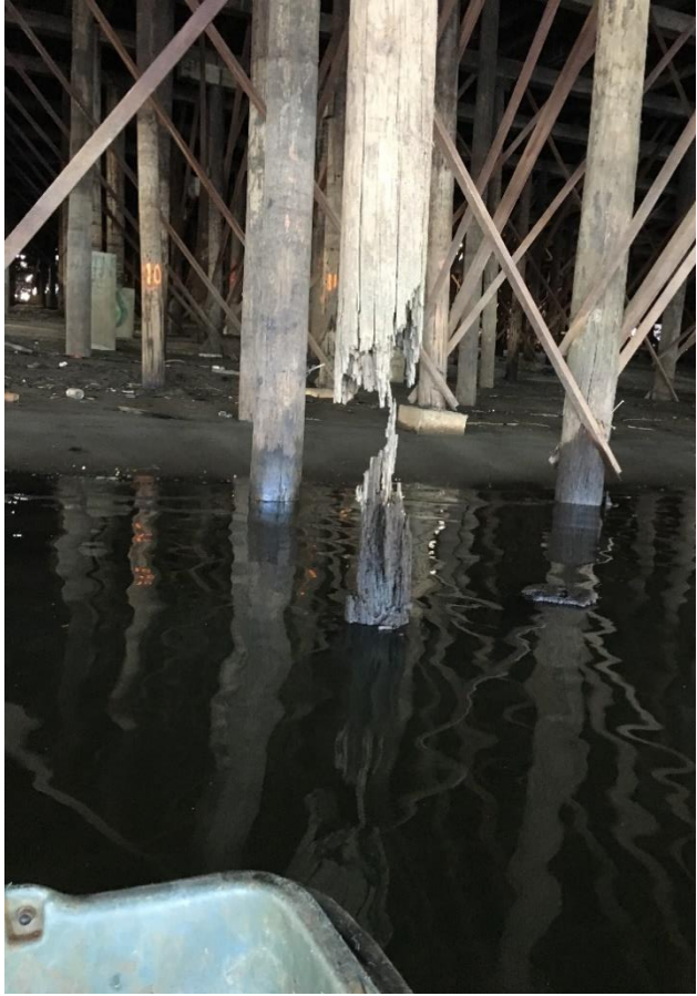
Photo #4 – Completely rotted pile
