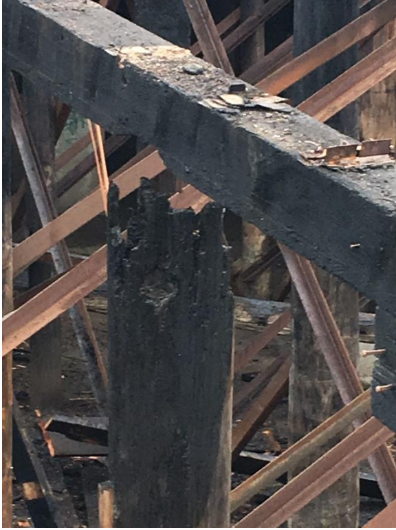
PHOTO NO. 9: Fire damaged pile with cap still in place above.
