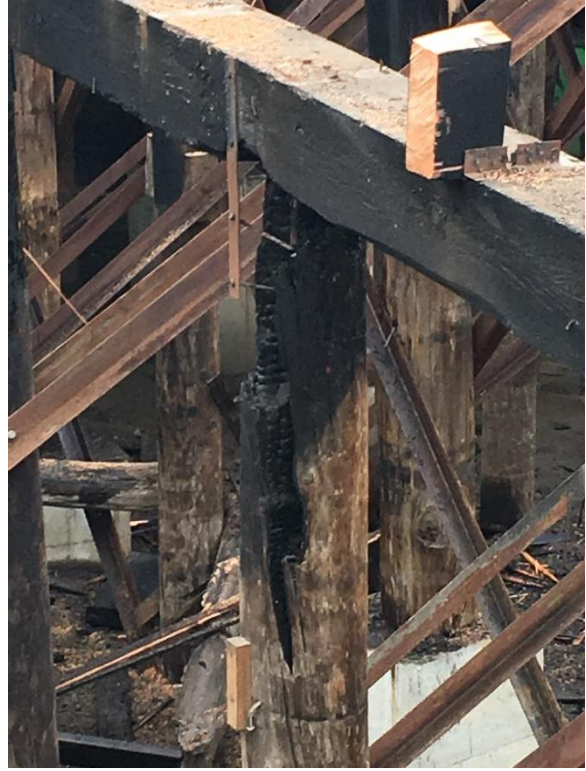
PHOTO NO. 10: Cap and stringers in place, but fired damaged pile below
