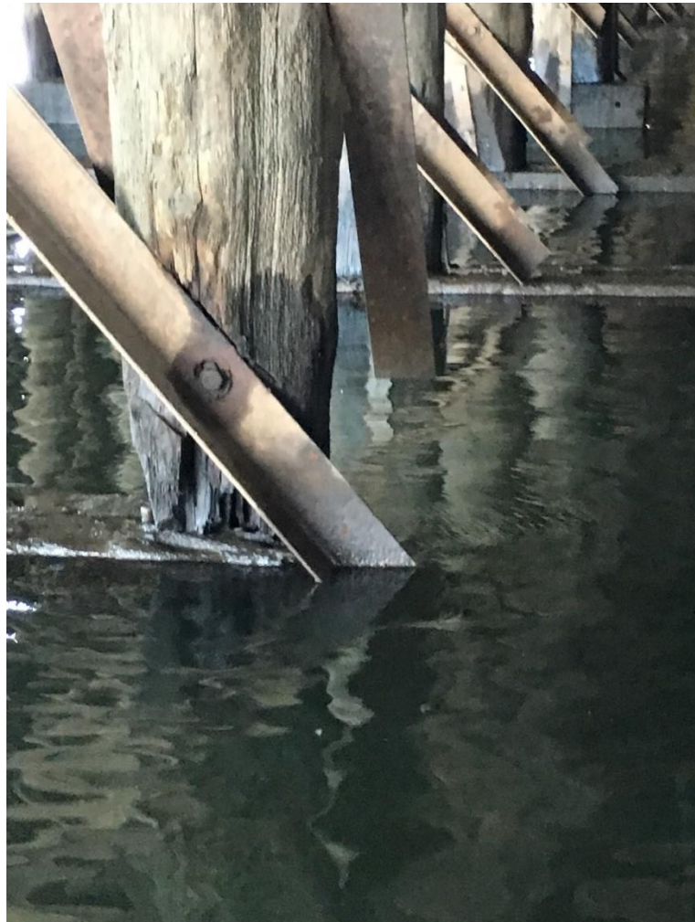
Photo #5 – Typical pile rot at waterline
