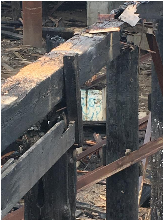
PHOTO NO. 7: Fire damaged piles and cap
