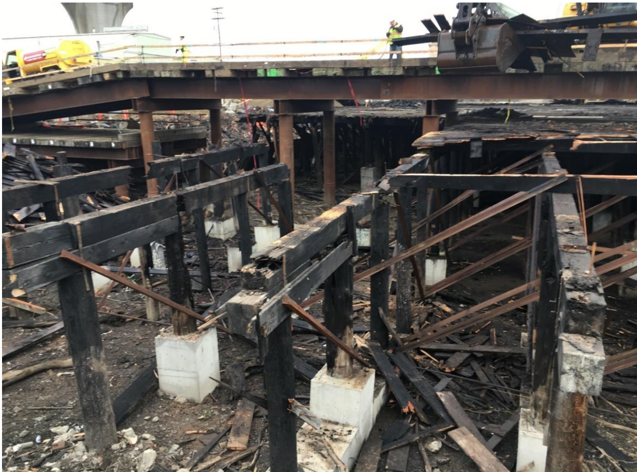
PHOTO NO. 5- Wharf area downstream of Access Trestle A with timber deck and stringers removed, exposing fire damaged piles and caps below.
