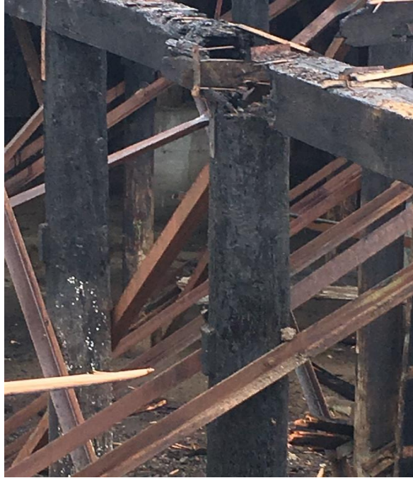
PHOTO NO. 6: Fire damaged pile cap with pile remaining.
