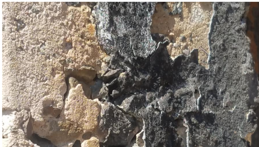
Photo 5 – Close-up of delaminating “tar like” material on wall surfaces within the structure.
