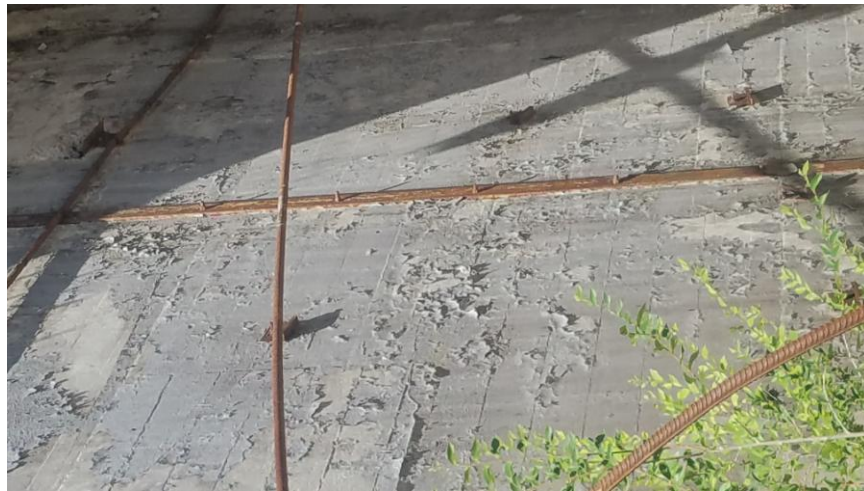
Photo 4 – Example of delaminating “Tar like” material on wall surfaces within the structure.
