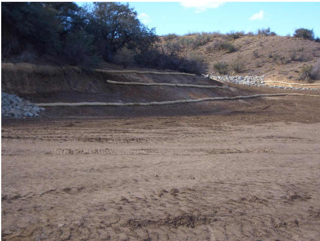
Final graded slopes with straw wattles
