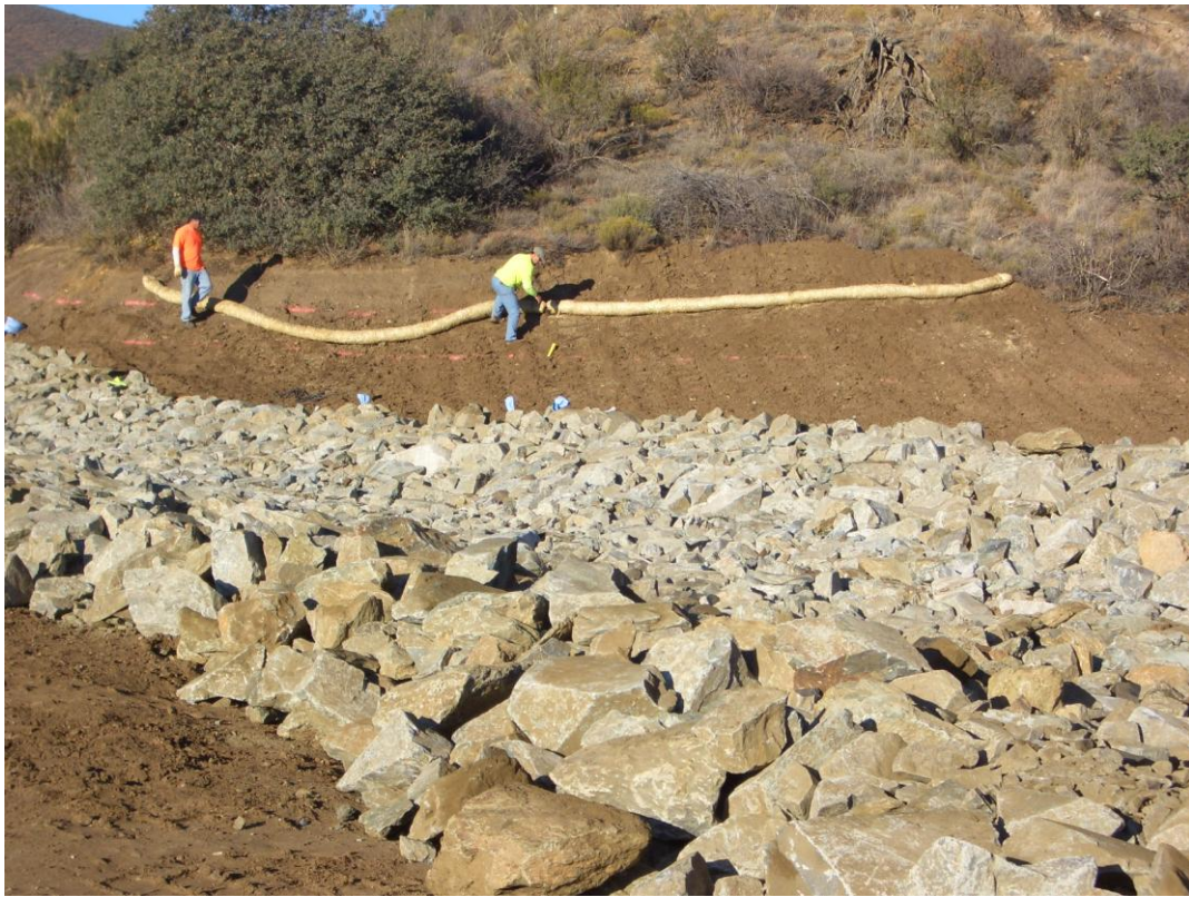
Installation of straw wattles along slopes
