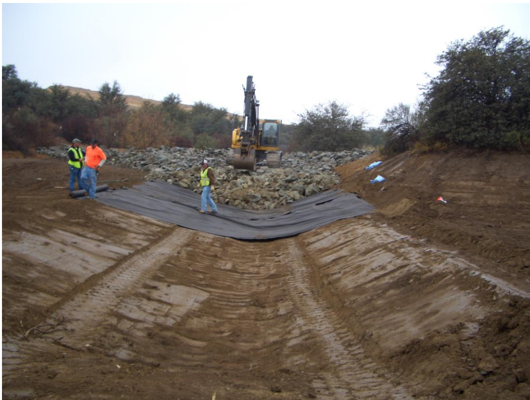
Diversion channel construction, downstream of NP area
