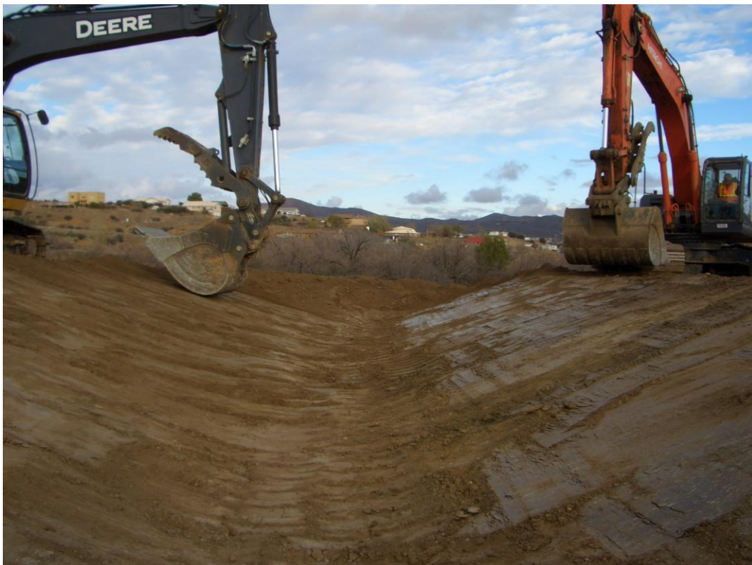
Diversion channel excavation and shaping
