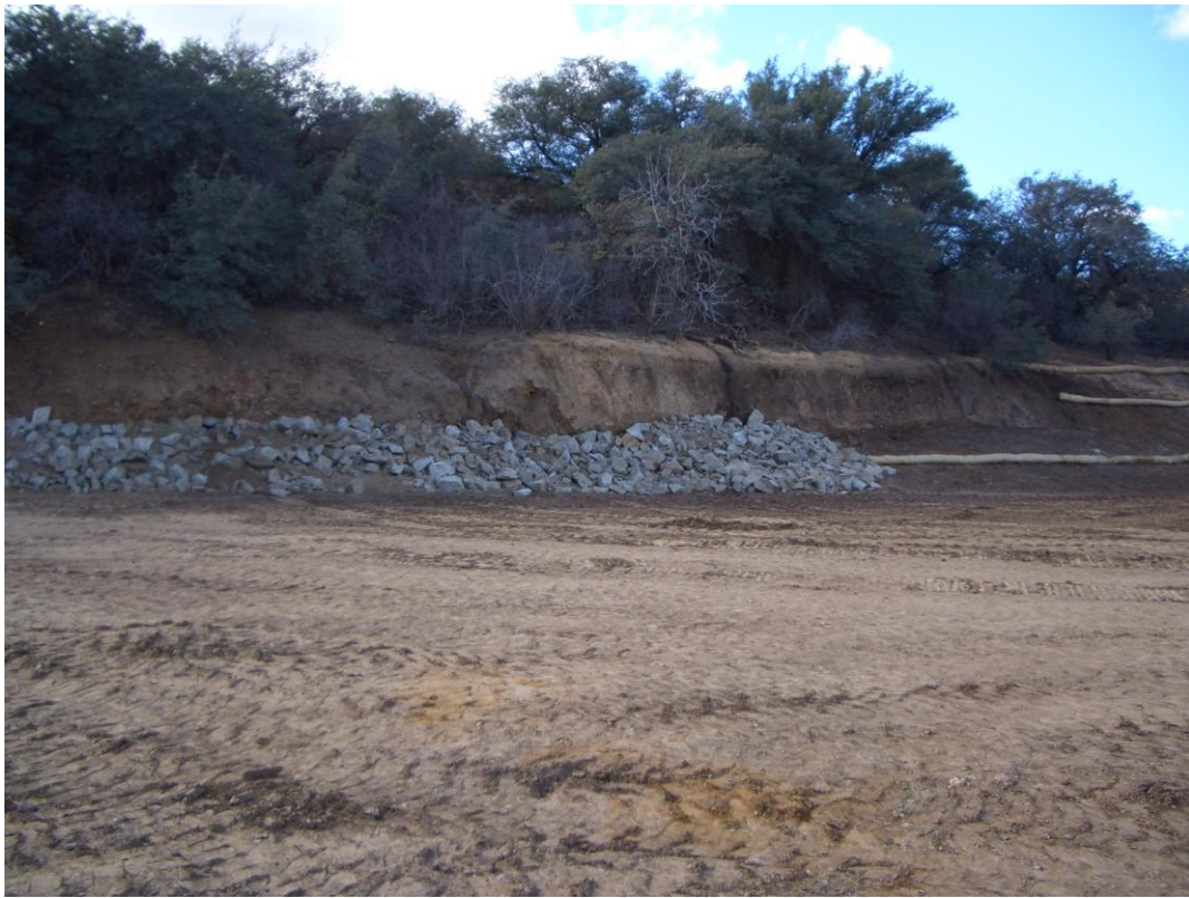
Vertical embankment with final riprap buttress
