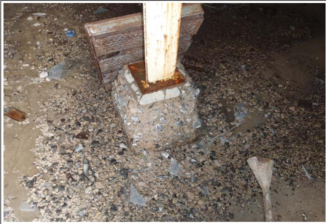
14. Corroded concrete pillars in Powerhouse Building #14
