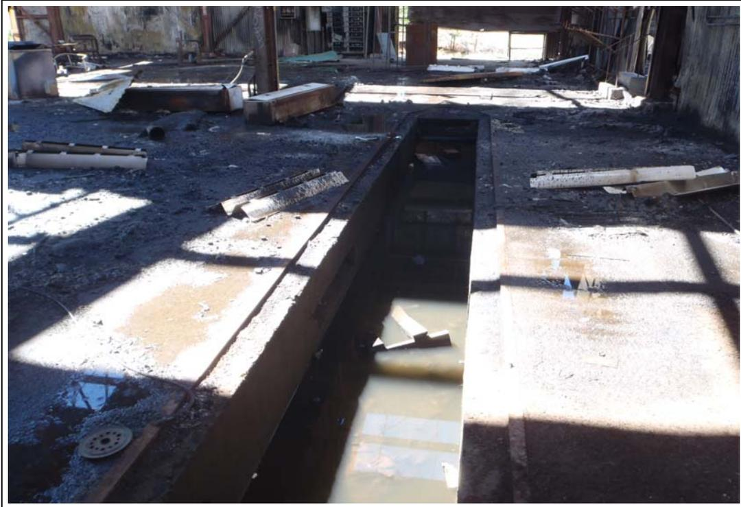
21. Vehicle maintenance pits in Warehouse Building #13 containing discolored water and debris
