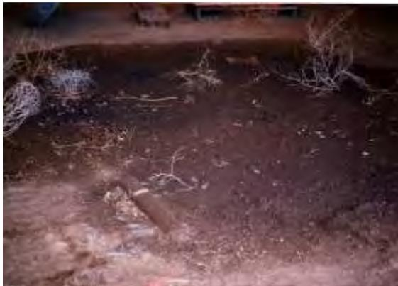
In the thirty-one buildings that were inventoried, NSP staff observed staining on the concrete floors. Dirt also covered the stained floors and exit areas used by vehicles. Stained concrete areas of the floor occurred because of leaking heavy equipment, discarded motor oil cans, and 5-gallon buckets used to store oily substances found in an upside down position.
