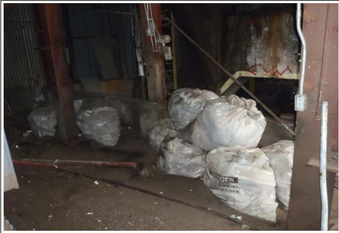
16. Bagged asbestos-containing materials (ACMs) on ground floor of Powerhouse Building #14
