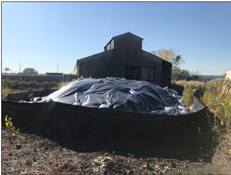
Photo #8: Looking south at Pile C (covered) with silt fence installed.
