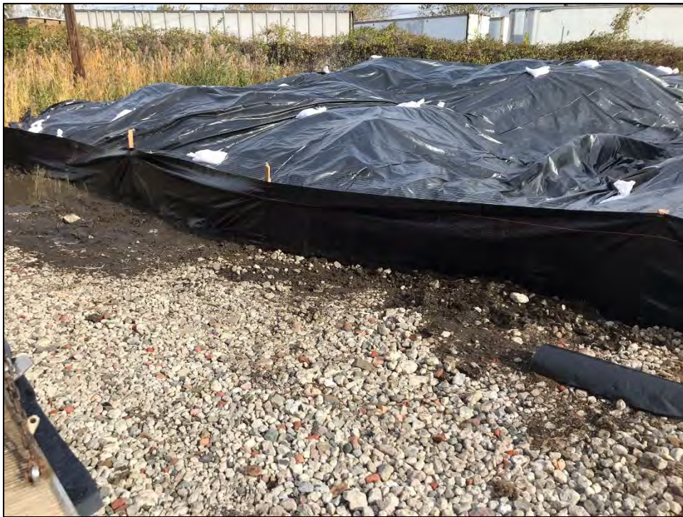
Photo #4: Looking NE at northern side of Pile A with silt fence installed.
