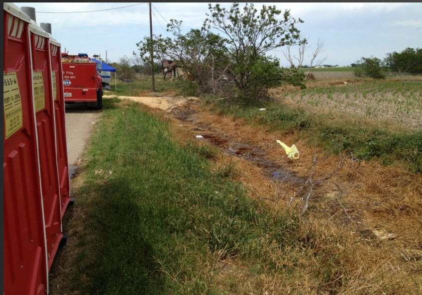
Contaminant pathway from explosion site. TCEQ berms ditch to restrict further flow.
