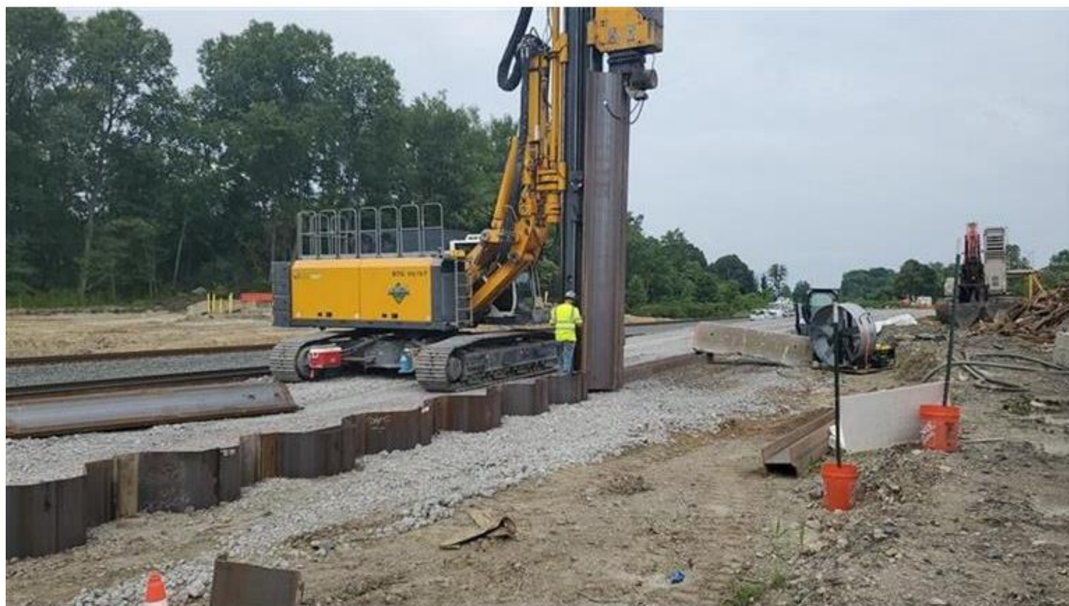
Sheet Piling in Car Scrapping Area 4, Facing Northeast
