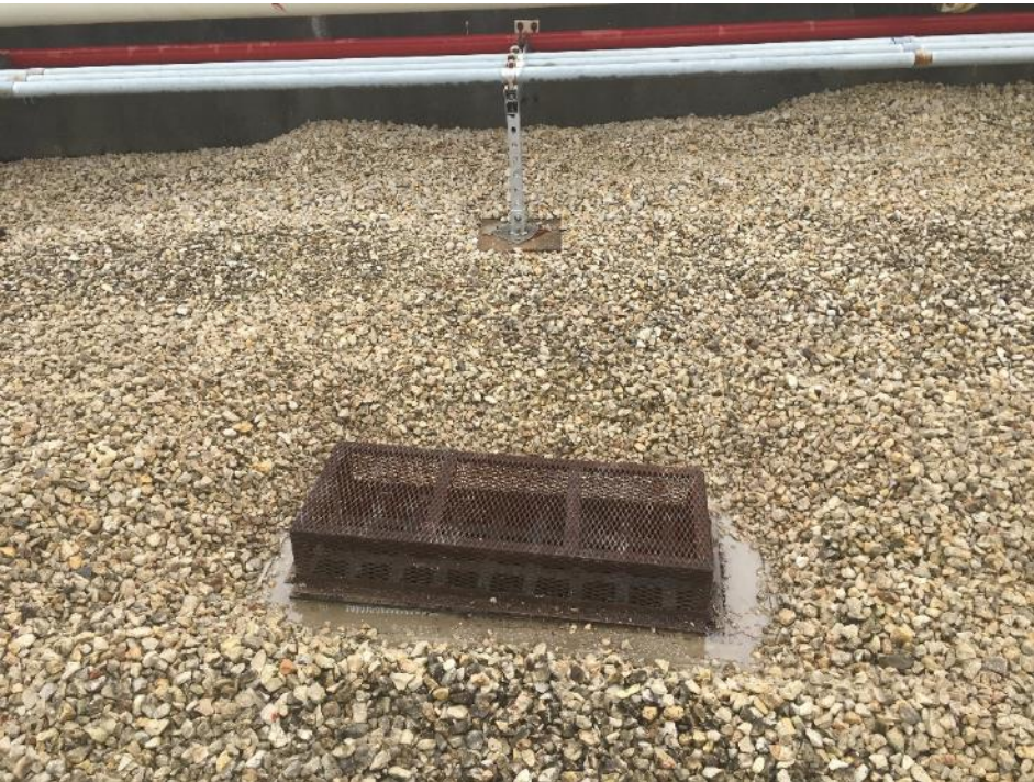
Primary Containment Drain
