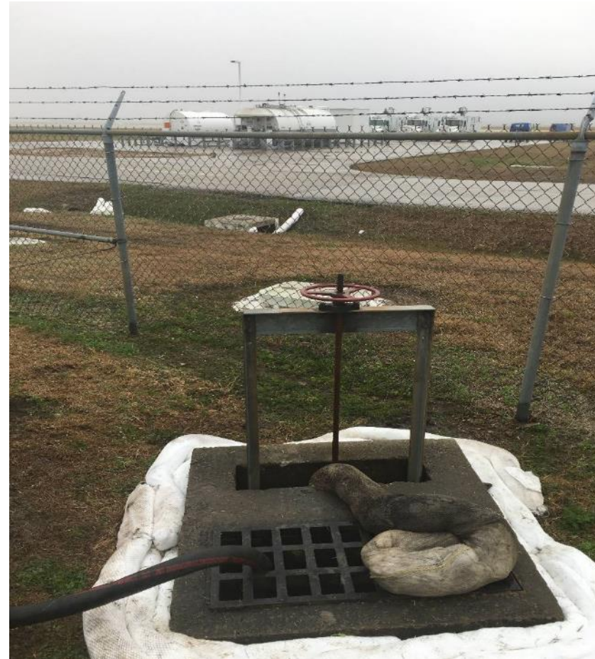
Sluice Gate Valve
