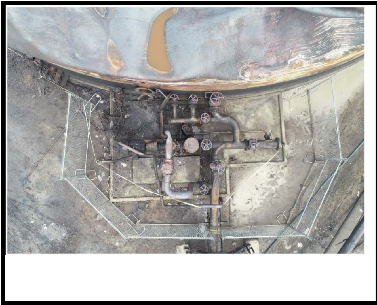
Overhead view of the Manifold and Associated Piping
